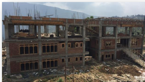
Figure 1: Package A Physical progress of Main Building
