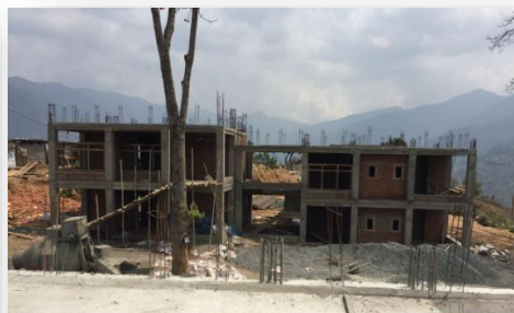
Figure 2: Package B Physical progress of Hostel Block
