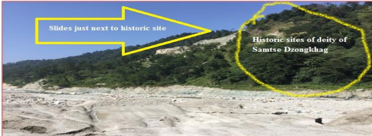
Figure (xxiii) - Slides and threat to historic sites (Along Dhamdum river few meters below suspension bridge), Samtse
