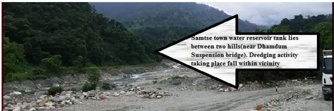
Figure-(x) Location of Water Tank (near suspension bridge Dhamdumriver), Samtse
