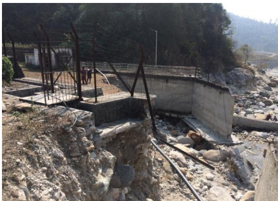
Figures- (xi) & (xii) RCC protection wall two panels and weir dam across Dhamdum stream located opposite to Suspension Bridge reported damaged by swollen river on September 25, 2018 and one main cause is due to river dredging down stream
