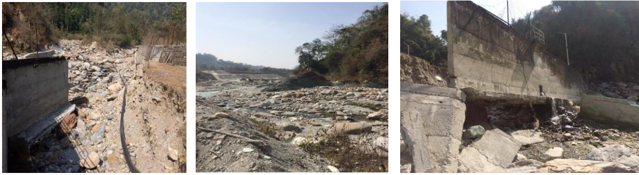
Figure (xii), (xiii), (xiv) and (xv) Major damage caused and maintenance awaited
