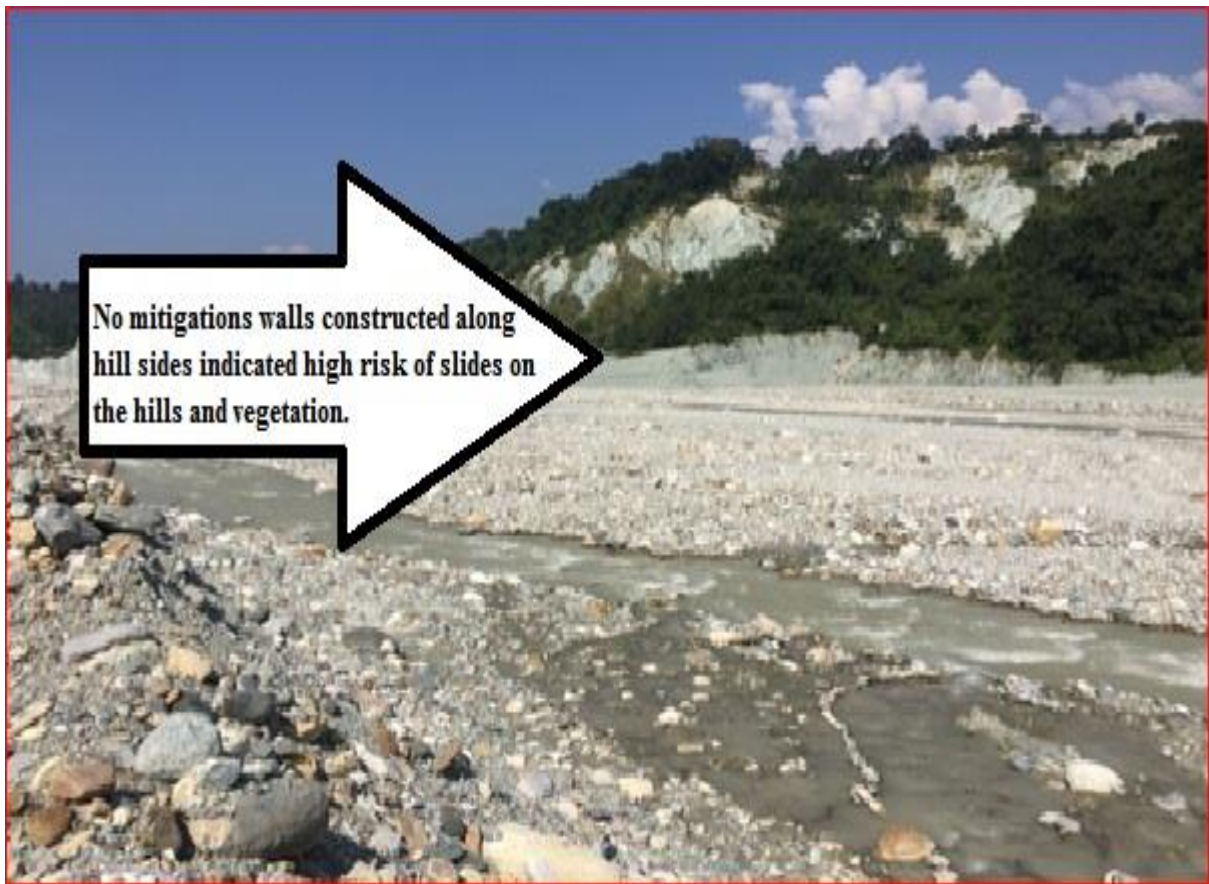
Figure (xxi) - scouring on the hill side
