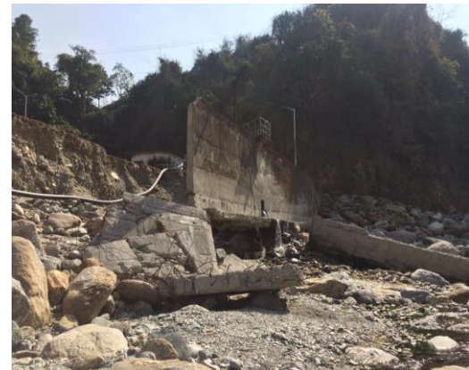
Figures- (xi) & (xii) RCC protection wall two panels and weir dam across Dhamdum stream located opposite to Suspension Bridge reported damaged by swollen river on September 25, 2018 and one main cause is due to river dredging down stream
