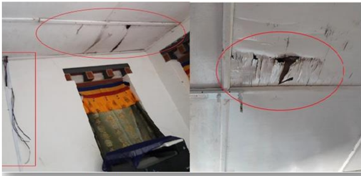
Figure 12. Damaged ceiling and electric wire at Useu and Samar CC
