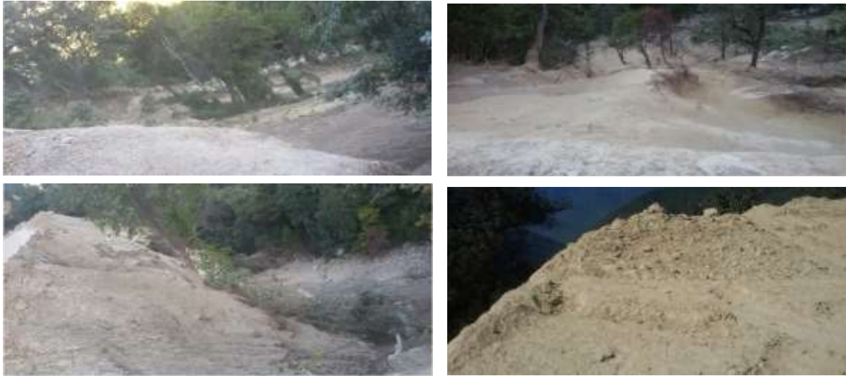
Fig: 2.17.11- Spoils materials dumped and freely rolled/pushed over the hill
