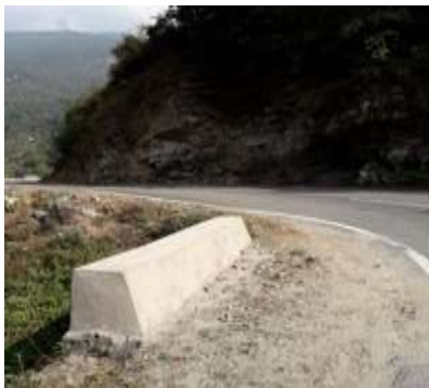
Repaired Parapets and RCC slab damaged by flash flood during monsoon season Culvert 12, Catch pit 4 Ch. 418 km as shown below.
