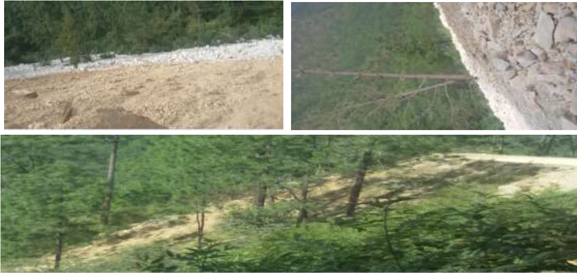
Fig.: 2.17.14- Freely rolled/pushed down of excavated materials over the hill
