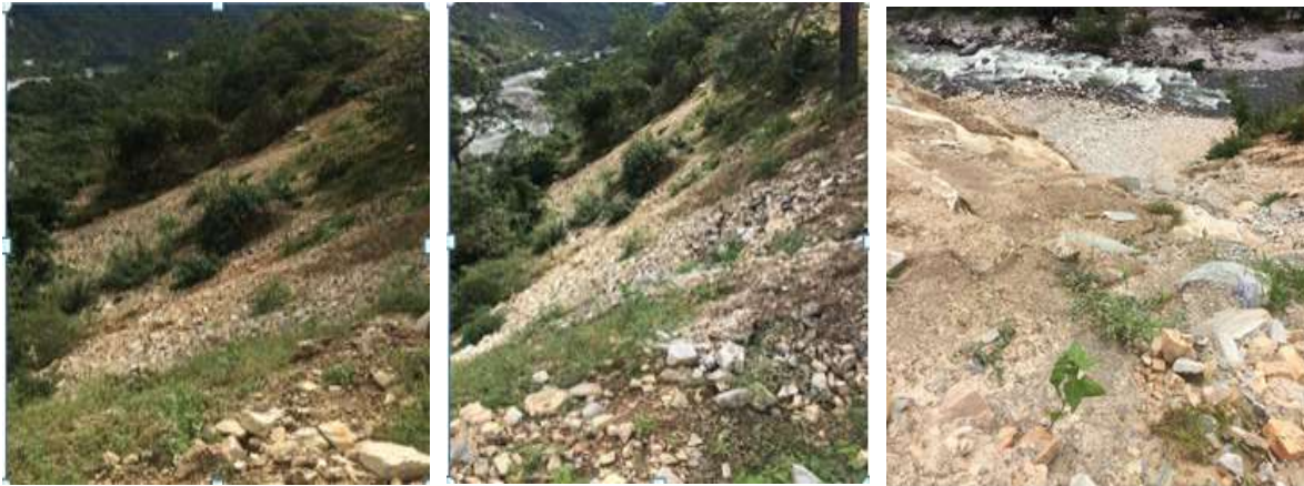
Fig: 2.17.15-Roll over of mucks over the valley
