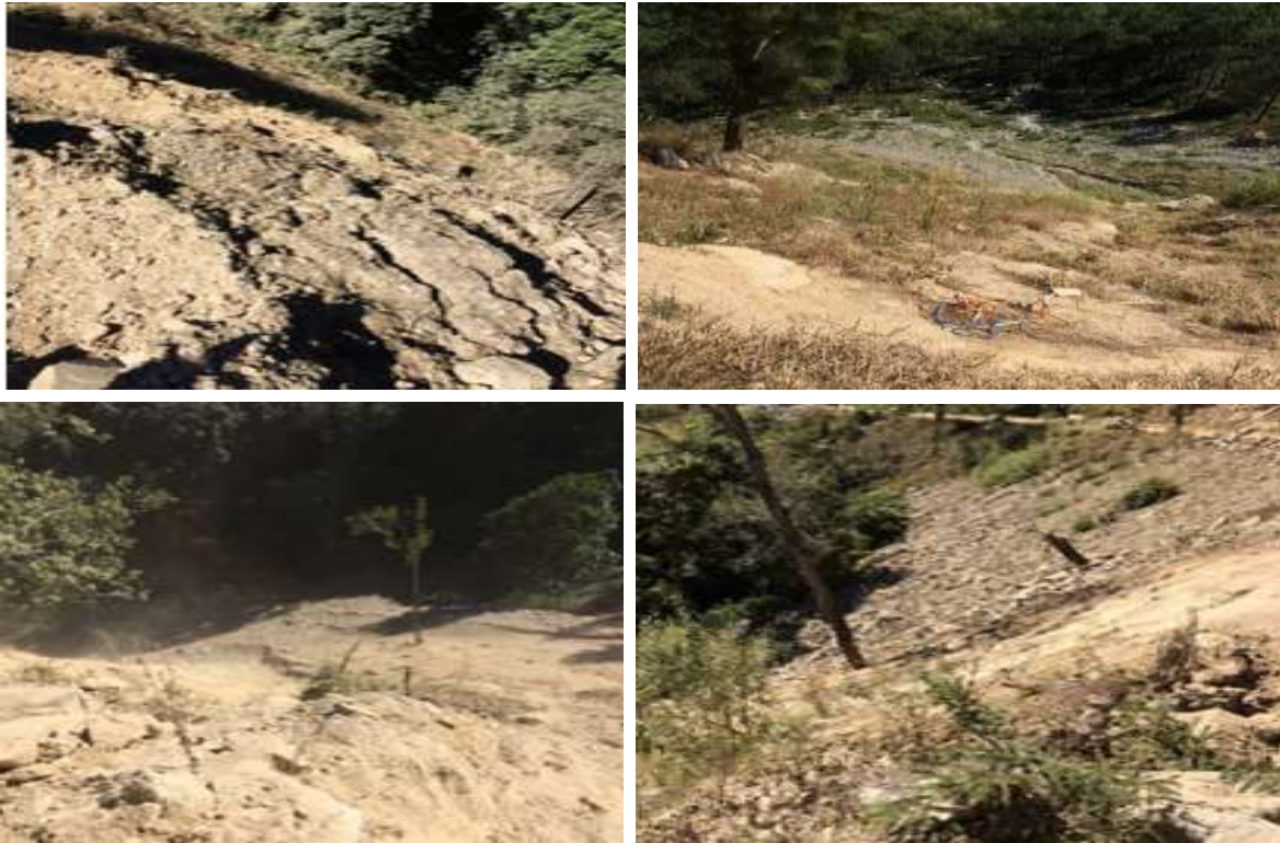
Fig: 2.17.16-Freely rolled/pushed down of excavated materials over the hill
