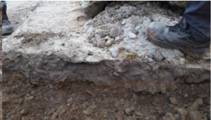
Section of L-drain without sub-base: Stone soling after the completion of Construction –noted during joint verification on 4.12.2017
