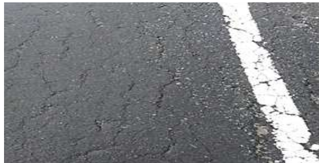
Fig: 12.2.1-Execution of Defective and substandard pavement works
