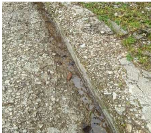
Fig:12.2(2)-Drain in dilapidated condition- cement plaster on plum concrete worn-out and exposing aggregate on the PCC
