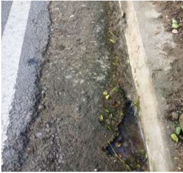
Figure 21.3: L-shaped drain PCC worn out
