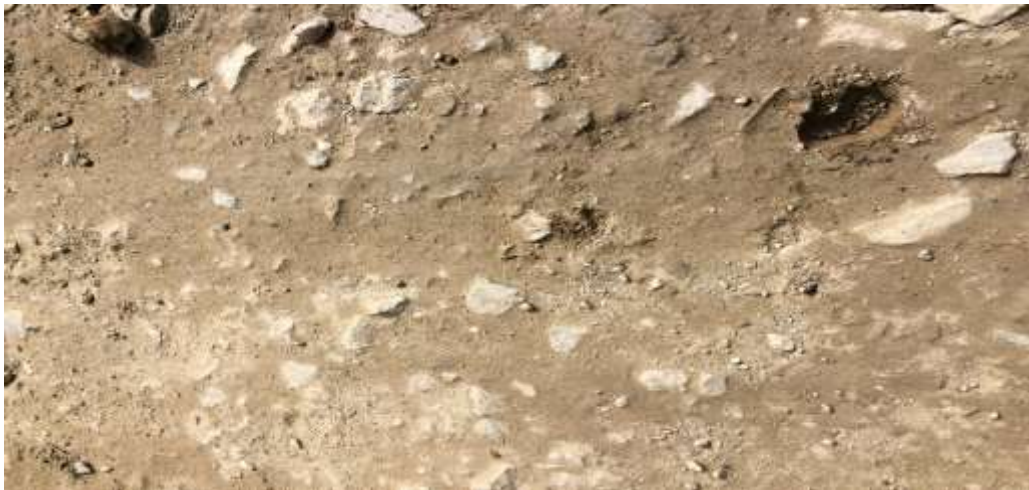
Fig: 14.3: Defective WMM works
