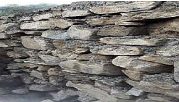
Fig: 12.2-Inferior masonry works
