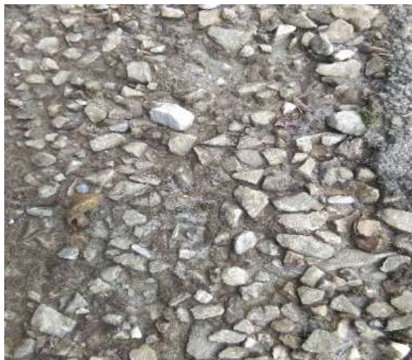
Fig:12.2(2)-Drain in dilapidated condition- cement plaster on plum concrete worn-out and exposing aggregate on the PCC
