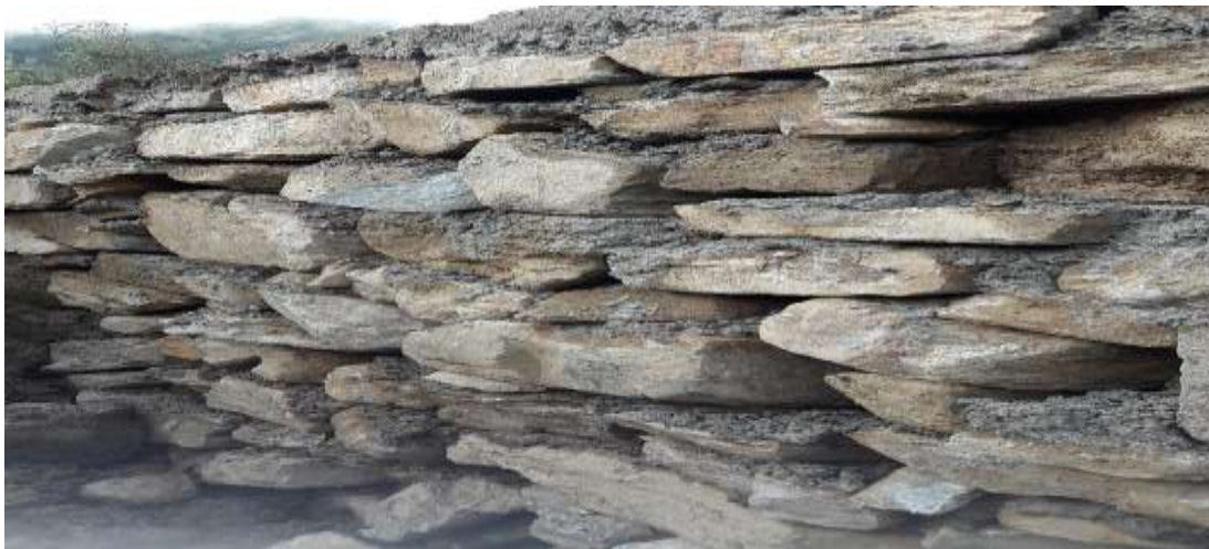
Fig: 5.1: Defective construction of CRM wall
