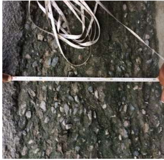
Fig:18.3: L-shaped drain measuring only 600mm width
