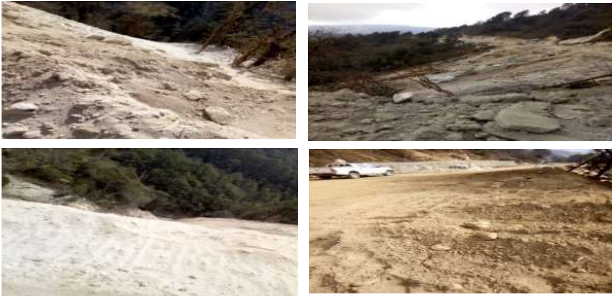
Fig: 2.17.8- Spoil materials dumped and freely rolled/pushed over the hill causing damaged to the environment
