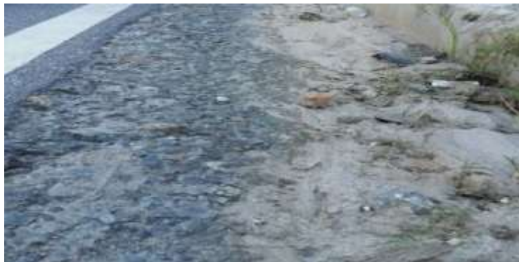
Fig:13.1- Defective drain work
