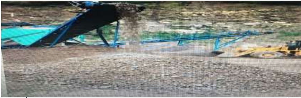
Picture showing crushing machine producing WMM material at site.
