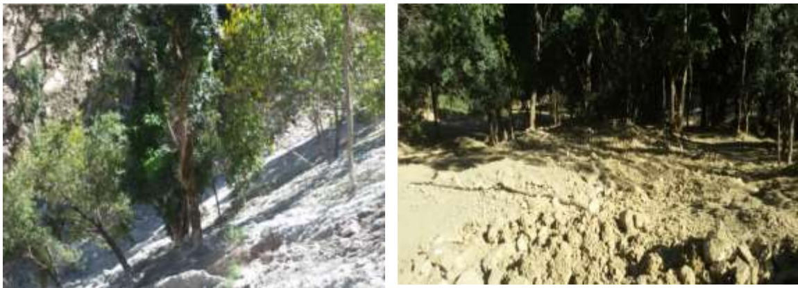
Fig: 2.17.12- Freely rolled/pushed down of excavated materials over the hill
