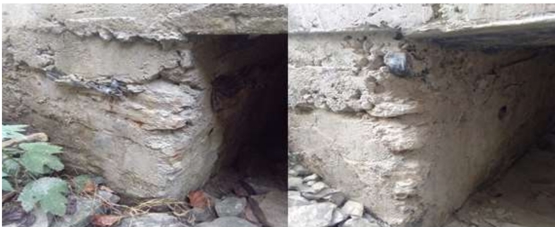
Picture 19.2: Sub-standard construction of CRM
