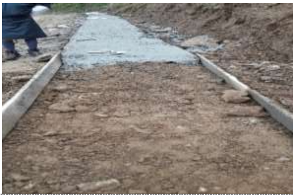
L-drain during construction without sub-base: stone soling as noted on 23.11.2017
