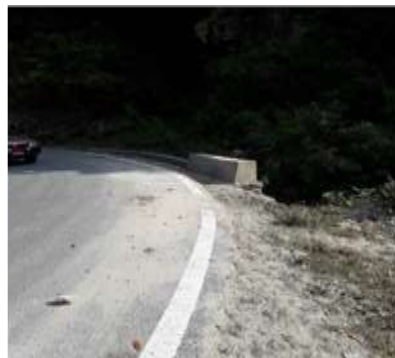
Repaired Parapets and RCC slab damaged by flash flood during monsoon season Culvert 12, Catch pit 4 Ch. 418 km as shown below.
