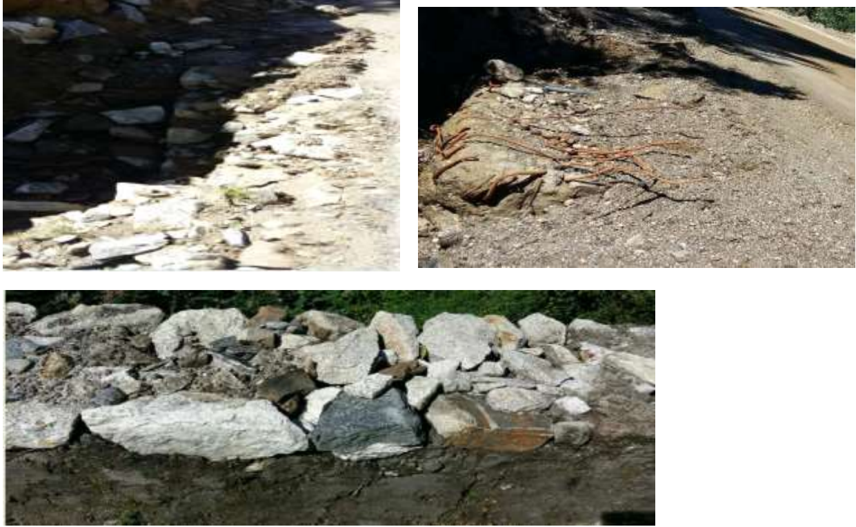
Fig: 15.1: Sub-standard RRM works
