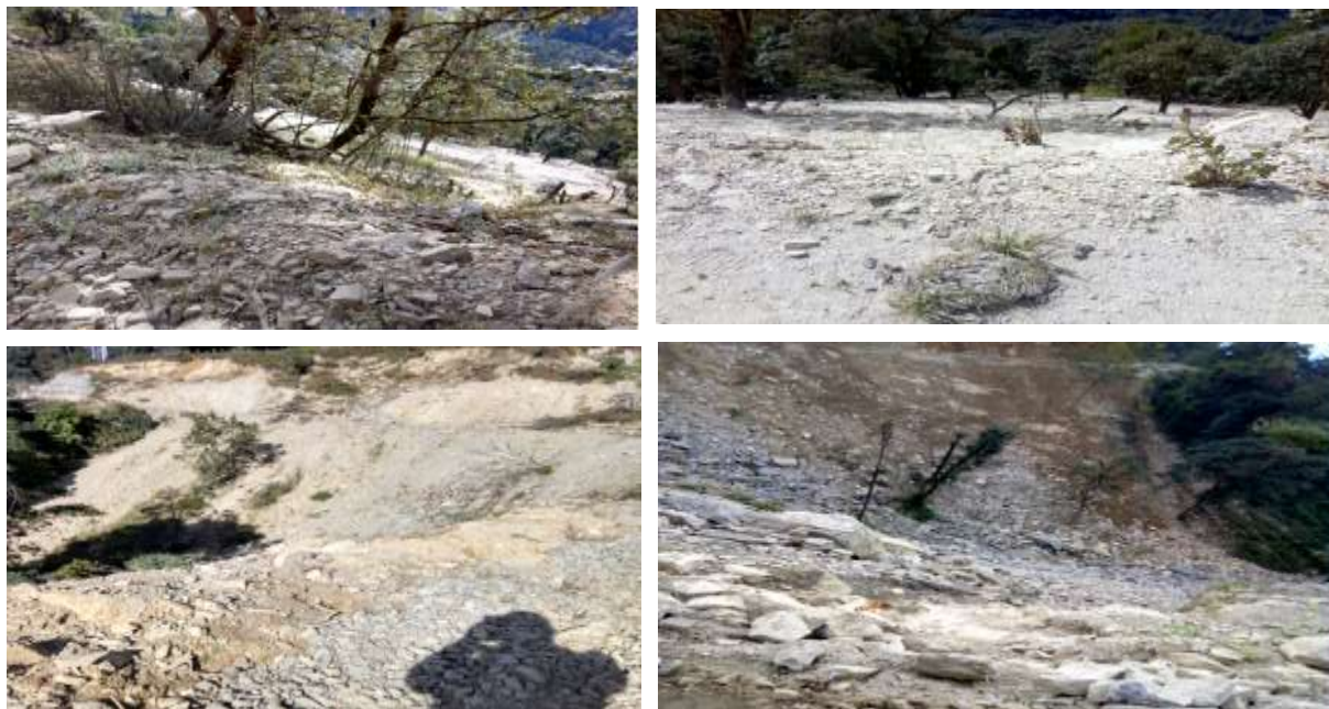
Fig: 2.17.10-Spoil materials dumped and freely rolled/pushed over the hill causing damaged to the environment
