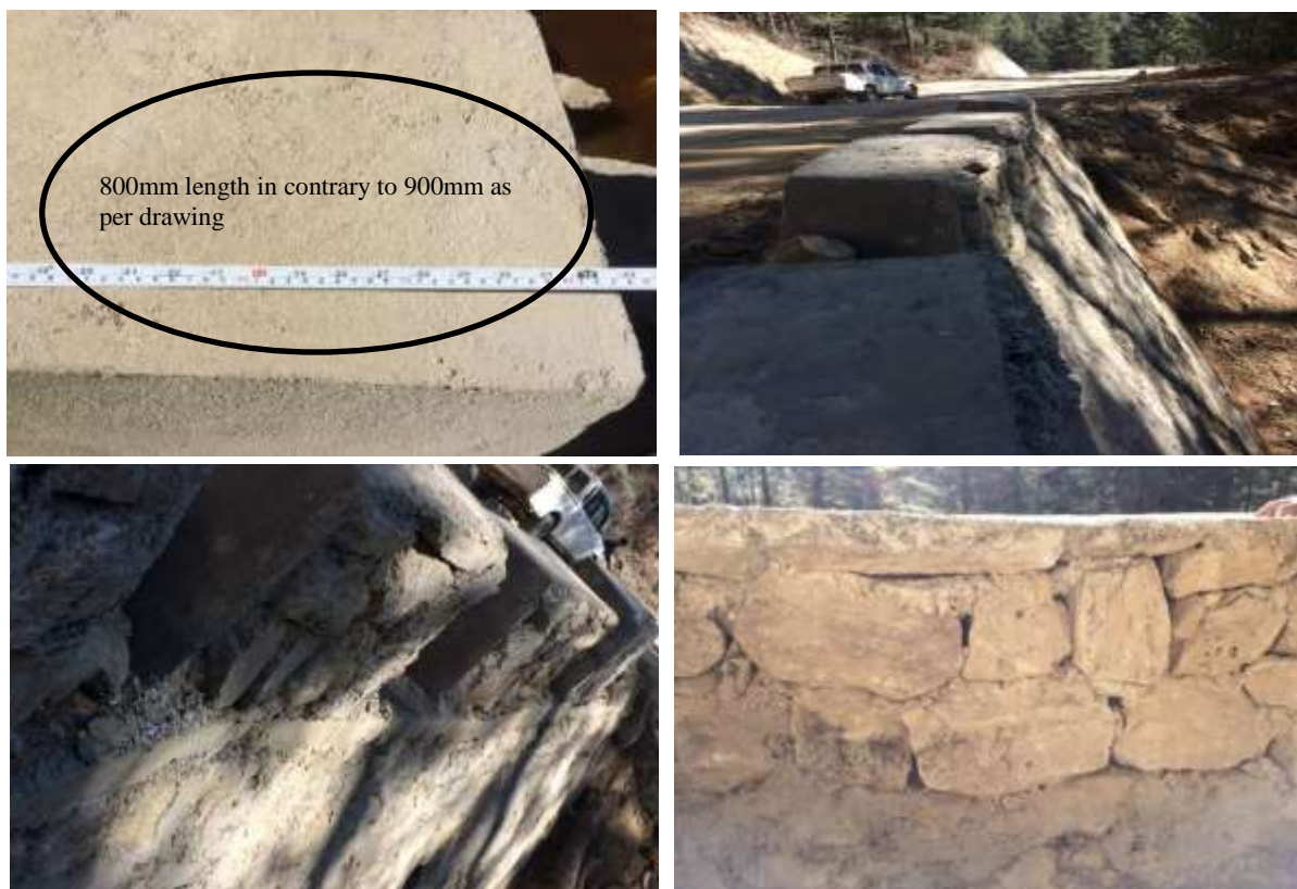
Fig: 14.4(1) - Construction of parapets not aligning to the specification
