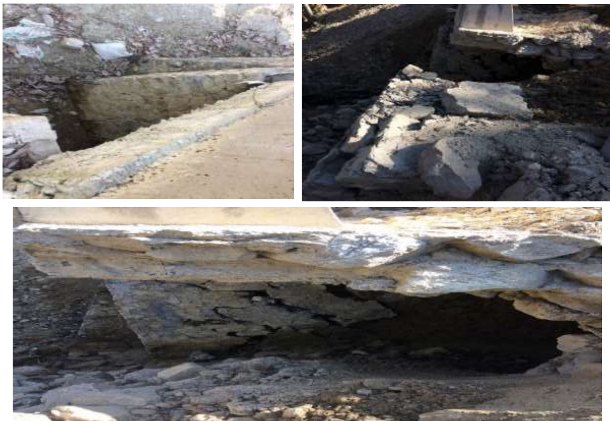
Fig:10.1 (1)- Damaged culvert
