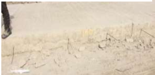
Fig: 21.1(2)- PCC block with 4 tie bars
