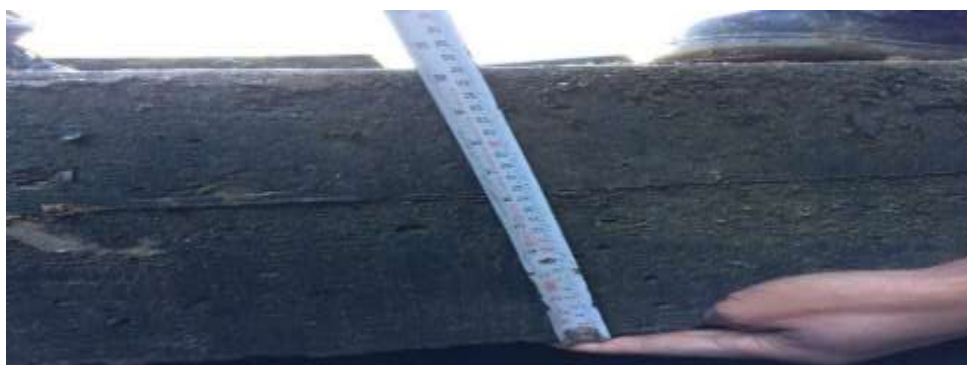
Fig: 7.3- 260mm thick deck slab
