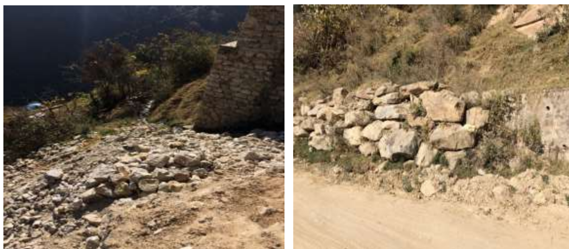
Fig:8.5- Damaged RRM walls
