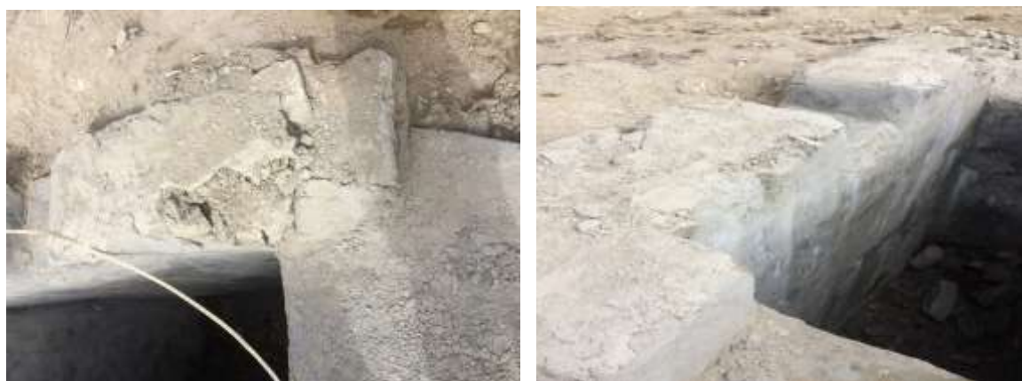
Fig: 12.1(1) - Damaged catchpits
