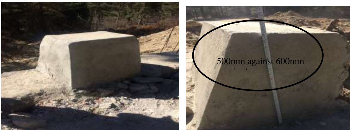
Fig: 14.4 - Construction of parapets not aligning to the specification
