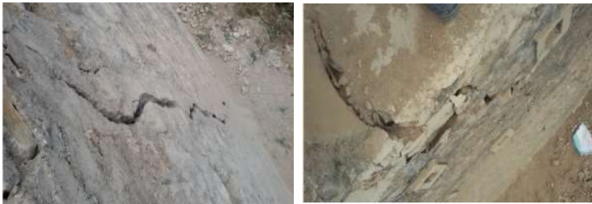
Fig: 9.1- Cracks developed in the Random Rubble Masonry walls
