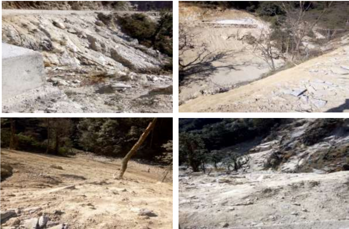
Fig: 2.17.2-Spoil materials dumped and freely rolled/pushed over the hill causing damaged to the environment
