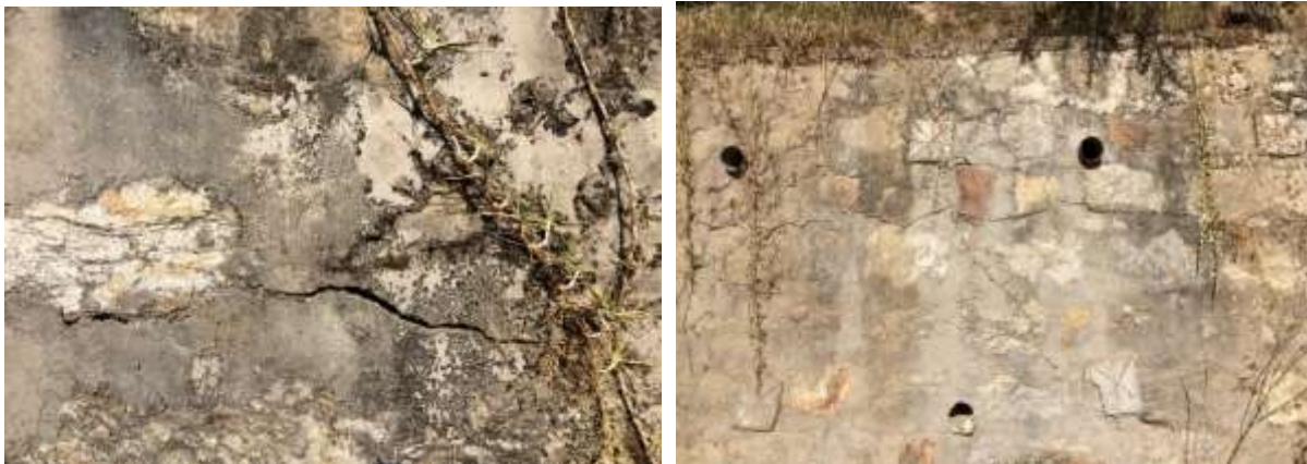
Fig: 8.5(1) - Cracks on RRM wall
