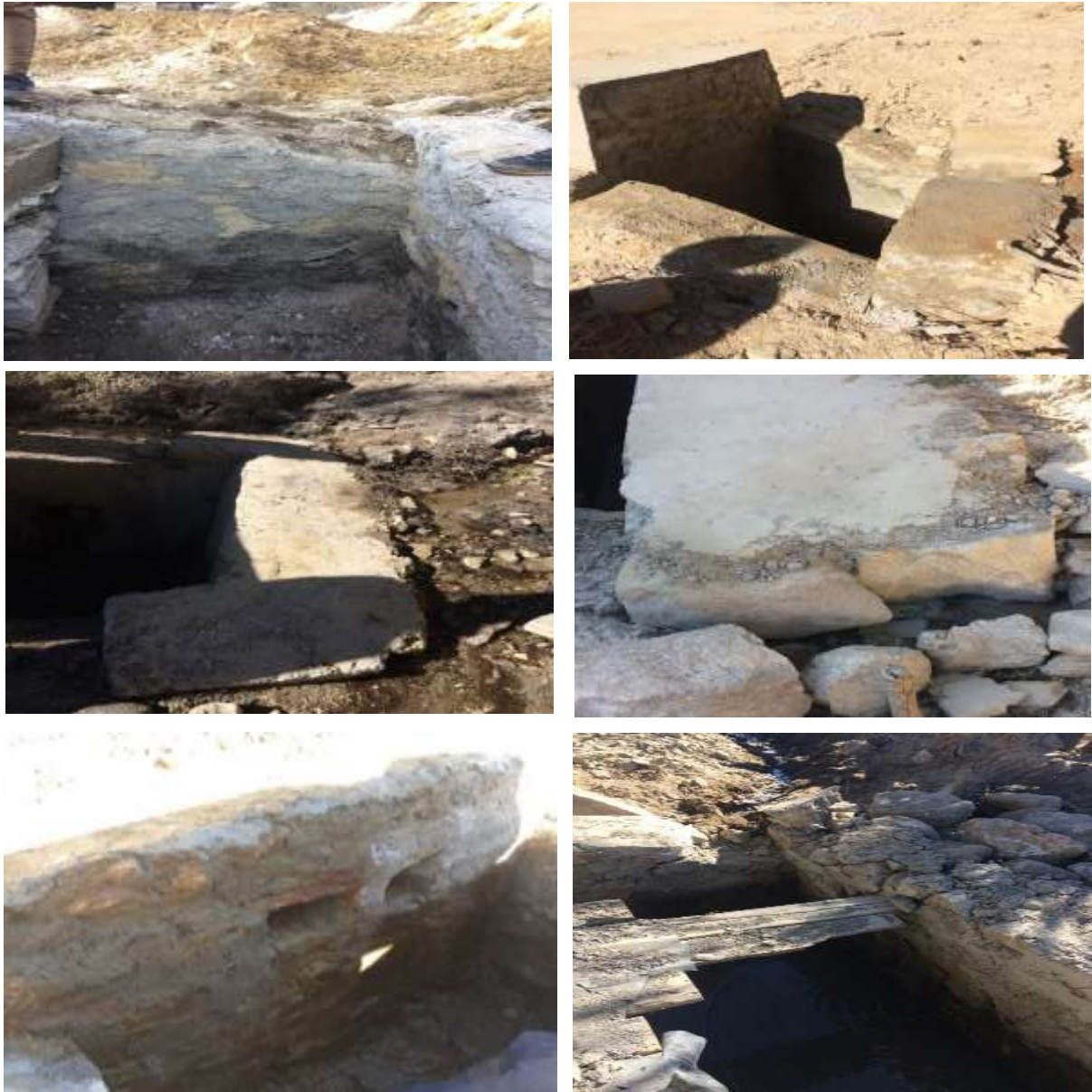
Fig.:14.2-Catch pit without opening leading to diversion of water along the roadside, which is completely deviating from the purpose of construction of catch pit and Catchpits not aligning to standard drawings and defective works
