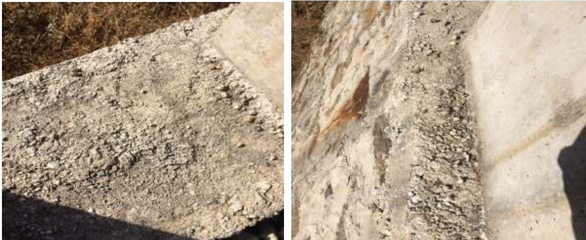
Fig: 18.2 - Defective PCC coping
