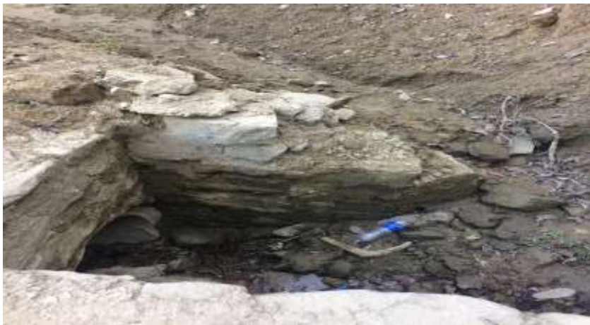
Fig: 5.1(a)- Sub-standard catch pit
