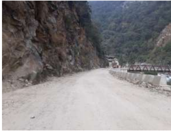
Para : 7.4-At end point Ch. 37,627 - 37,710 showing FC avoided with construction of R/Wall
