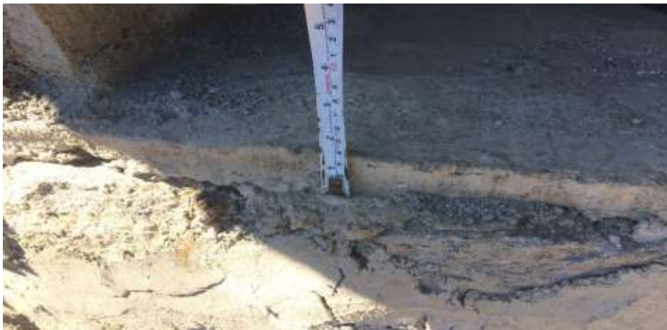
Fig: 14.1- PCC coping of 40mm done against 75mm requirement
