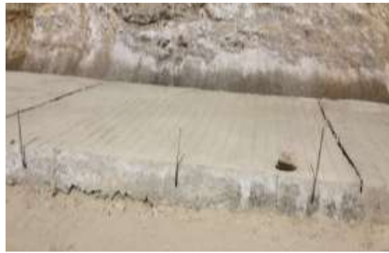
Fig: 21.1- PCC block with irregular center-to-center distance maintained
