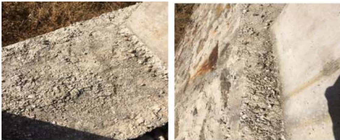
Para : 8.2-- Defective PCC
