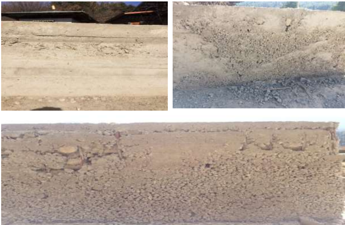
Fig:23.3- Defective Kerb Beams
