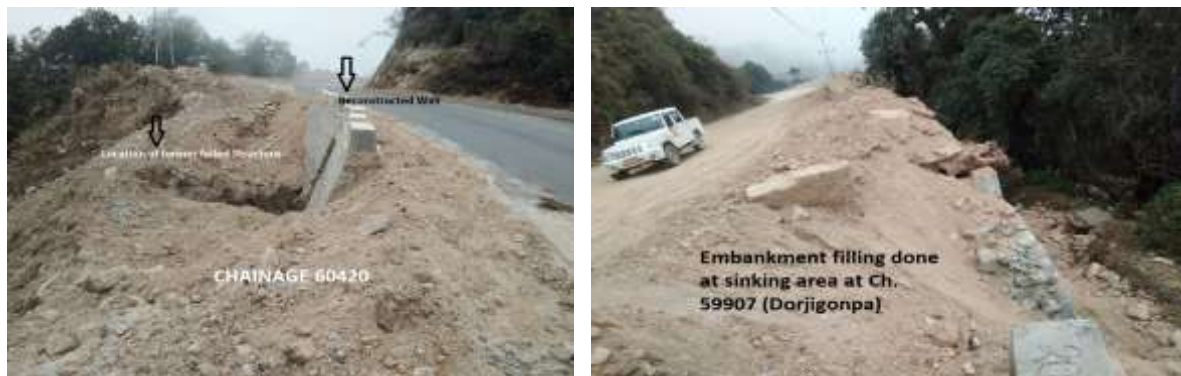
Para 11.1- Filling done at sinking area
