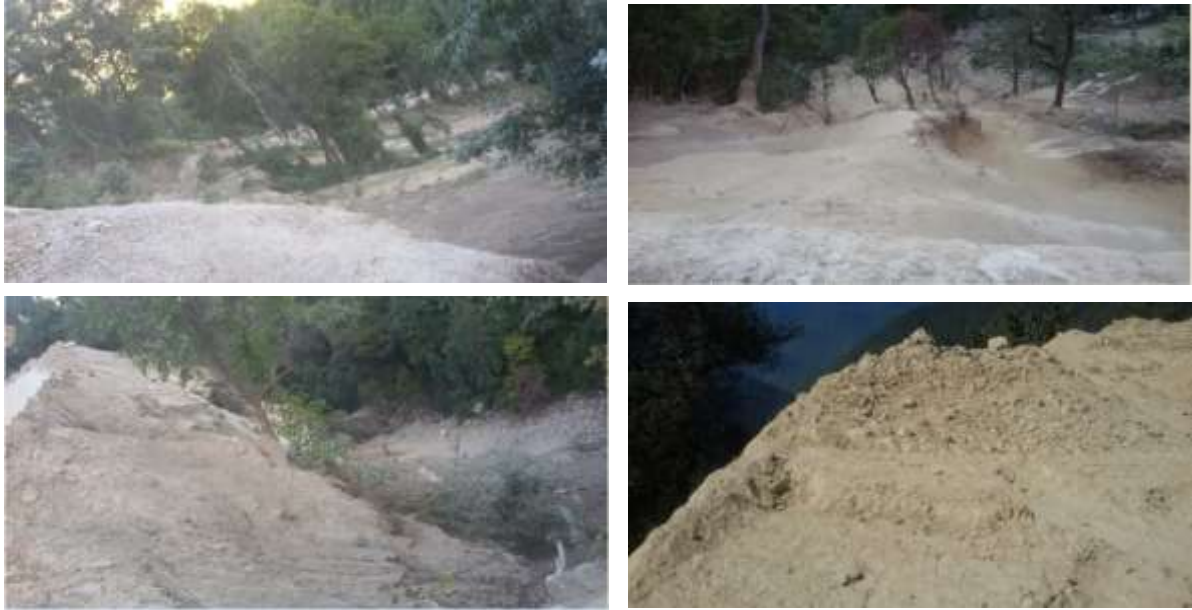
Fig: 2.17.11- Spoils materials dumped and freely rolled/pushed over the hill
