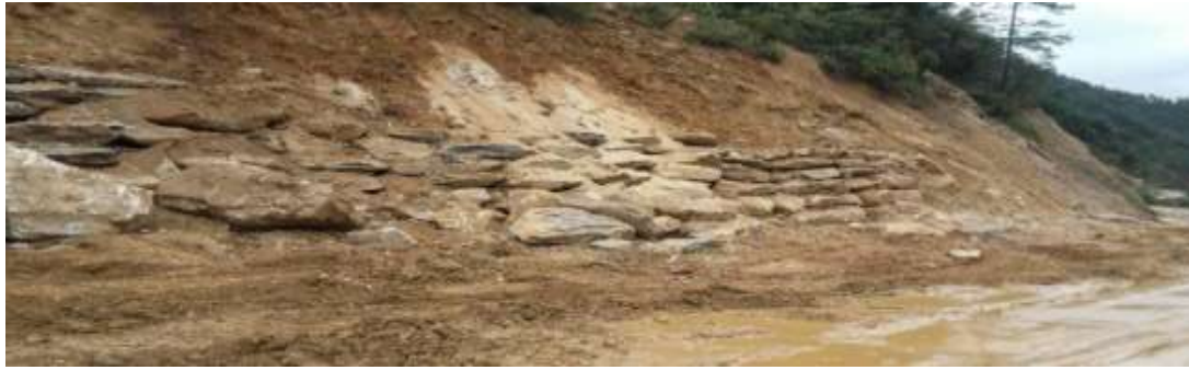
Para: 3.2(2)- Boulder Wall Construction
