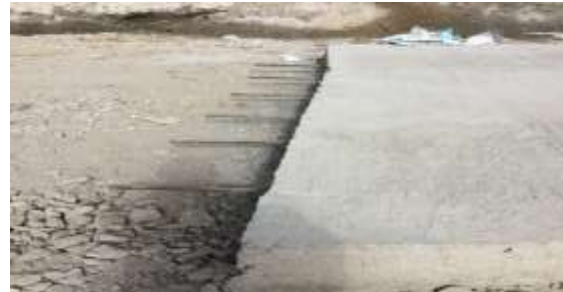
Fig: 21.1(3) Improper formworks leading to irregular PCC block
