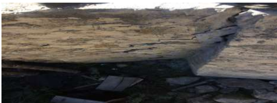
Fig: 7.1(2)- Damaged Wall
