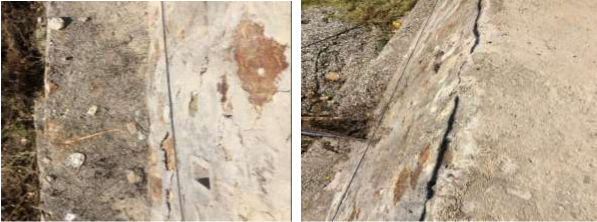
Fig: 8.4(1)-- PCC coping not done
