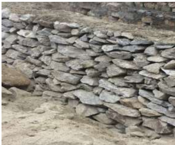
Fig: 2.5- Abutment walls constructed with huge boulder
