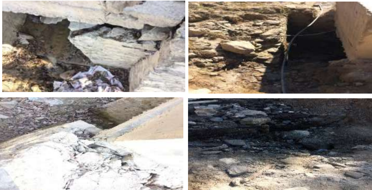
Fig:10.1- Damaged culvert
