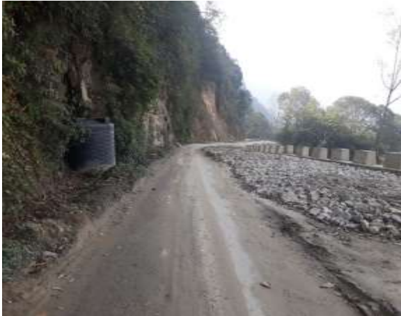
Para: 7.4-At Starting point Ch. 32000 m – 32053 m showing FC avoided with construction of R/Wall
