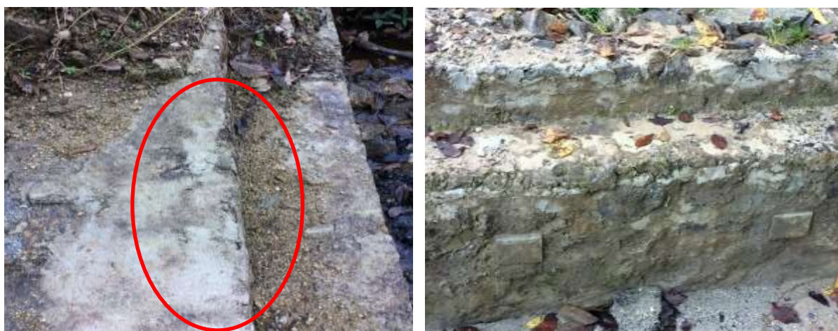
Fig: 7.2(1)- RC wall without PCC 1:3:6
