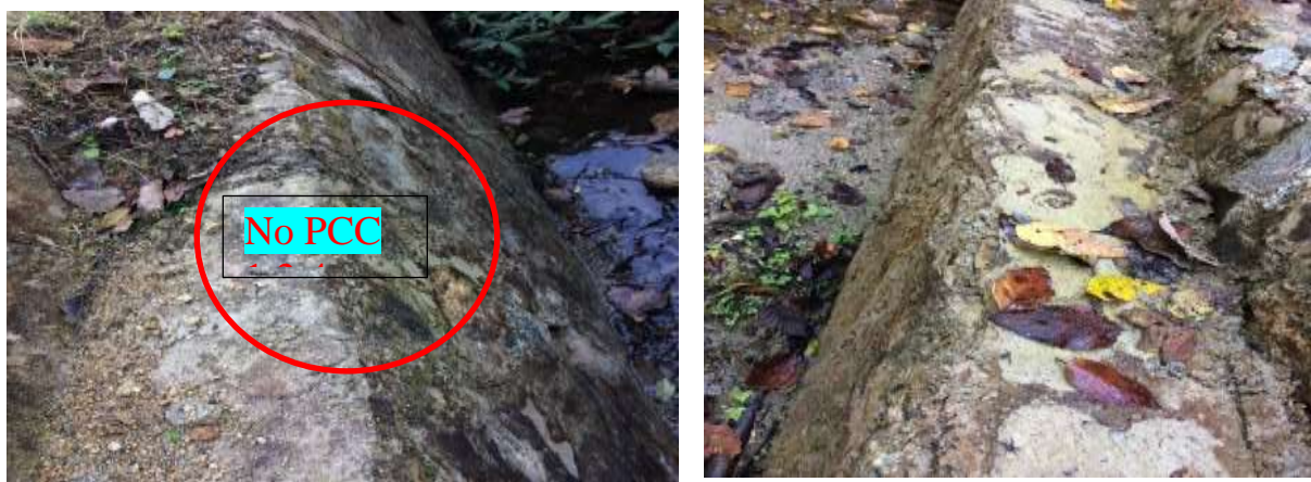
Fig: 7.1(1)- Abutment walls without coping
