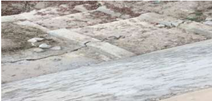
Fig:11.1(1) - Damaged RRM step walls
