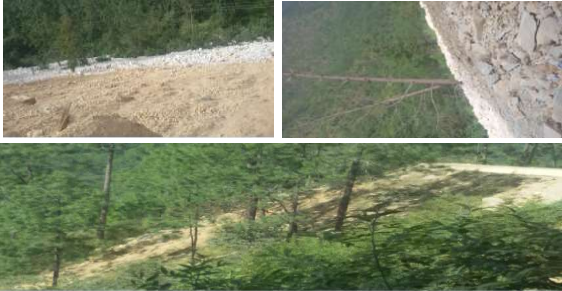
Fig.: 2.17.14- Freely rolled/pushed down of excavated materials over the hill
