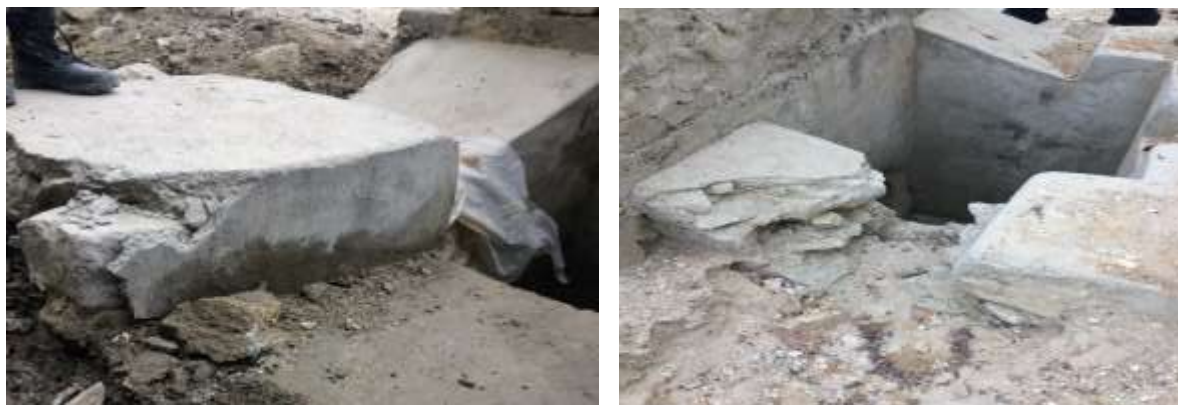
Fig: 12.1- Damaged catchpits
