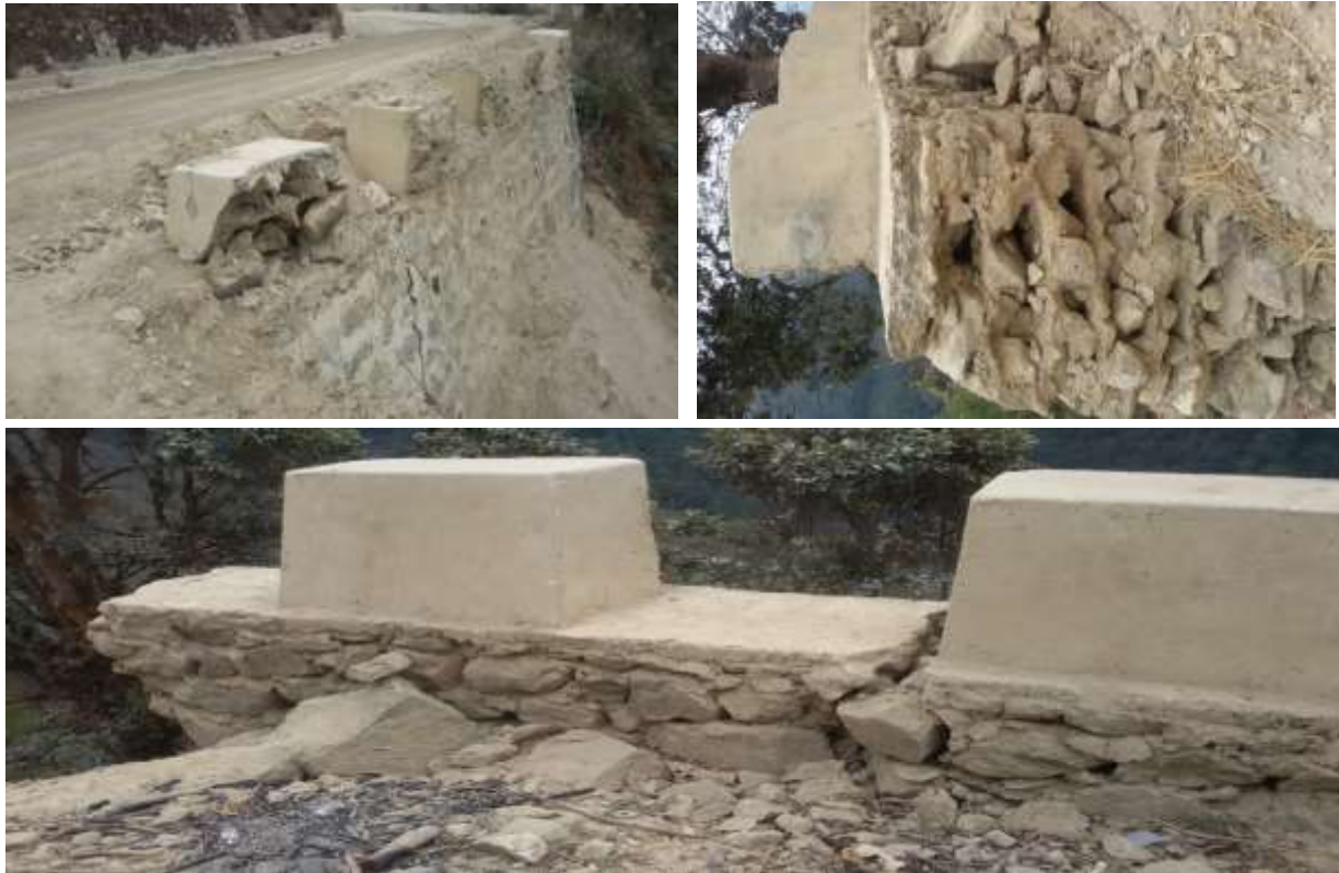
Fig: 9.1(1) - Collapsed RRM wall and sunk from the normal level of road
