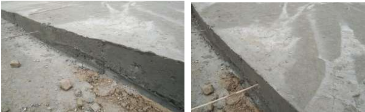
Para : 21.1-[Before and after pic showing that tie bars are re-inserted]
