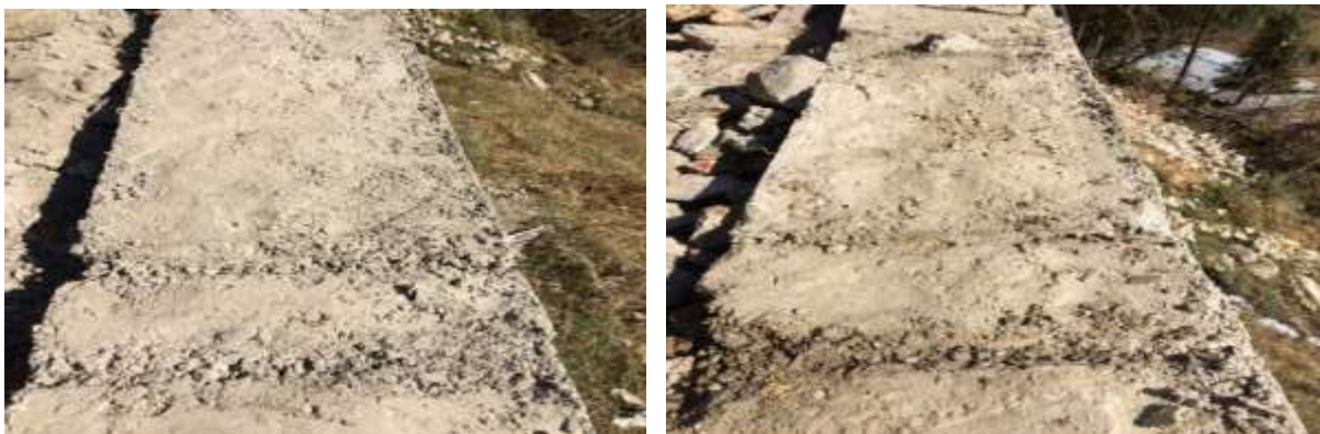
Fig : 8.4- Segregation of PCC
