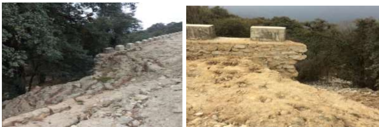
Fig:11.1- Damaged RRM walls at various chainages
