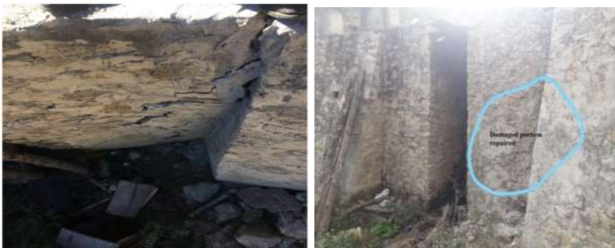
Para: 7.1- After Rectification
