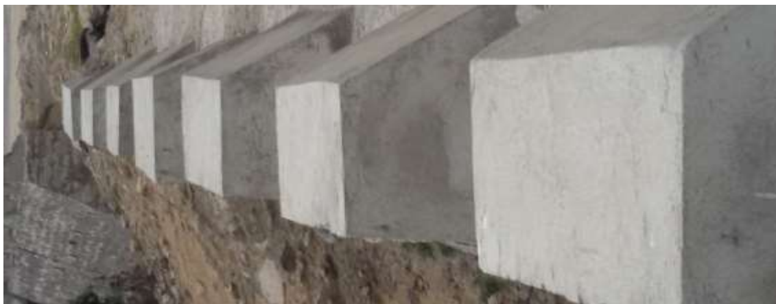
Fig: 9.2(1)- Parapets in irregular shape and improper finishing on back side of the parapets
