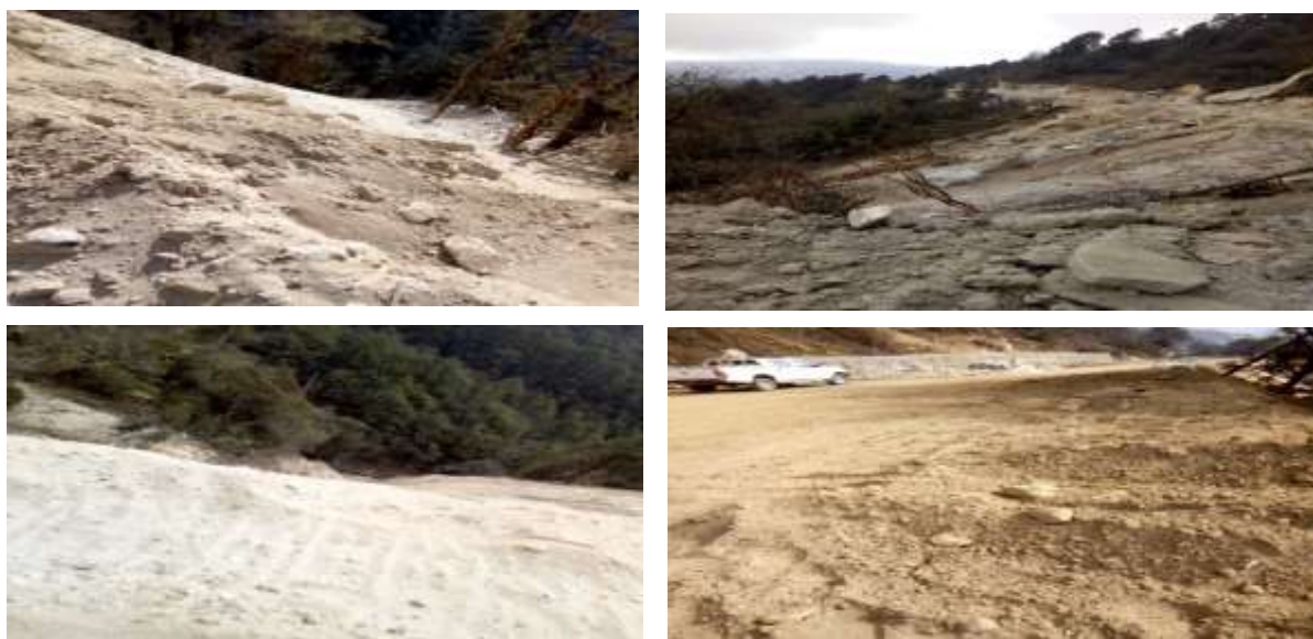
Fig: 2.17.8- Spoil materials dumped and freely rolled/pushed over the hill causing damaged to the environment
