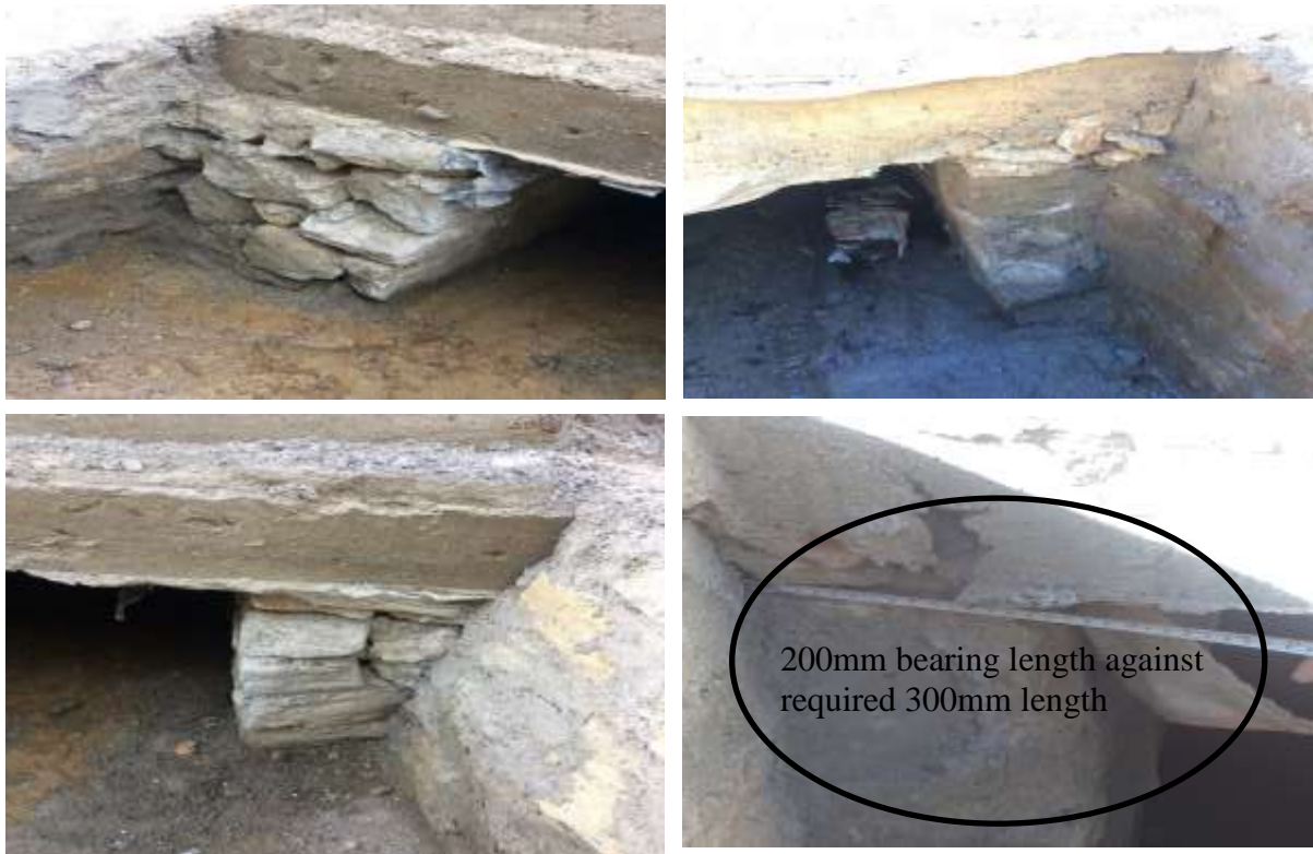
Fig:b14.3- Defective construction of culvert
