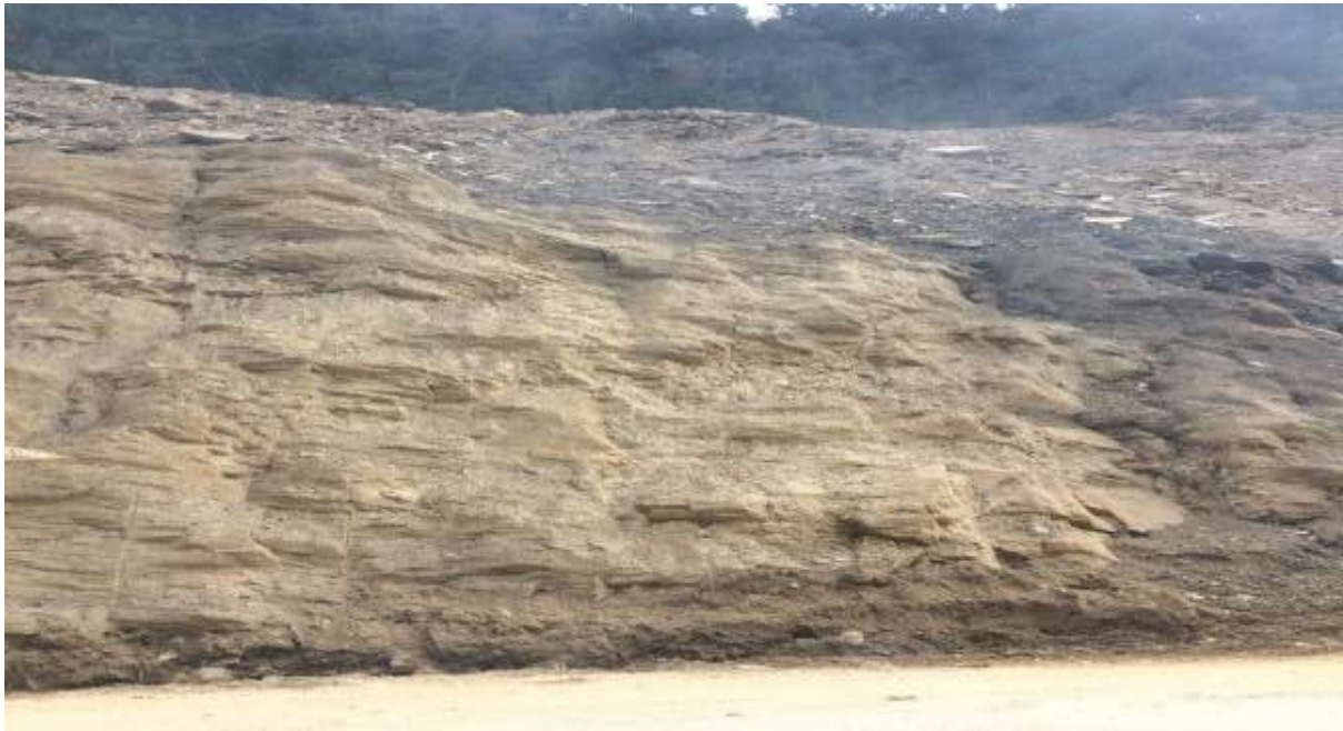
Fig: 31.2- Detailing excavations in deviation to designs and drawings
