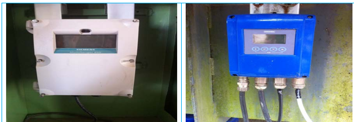
Figure No. 11: Defunct bulk meter at Jungshina and Dechencholing Treatment Plants
