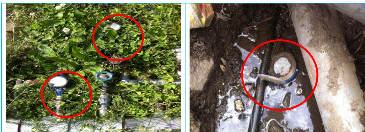
Figure No. 13: Inappropriate water meter installation
