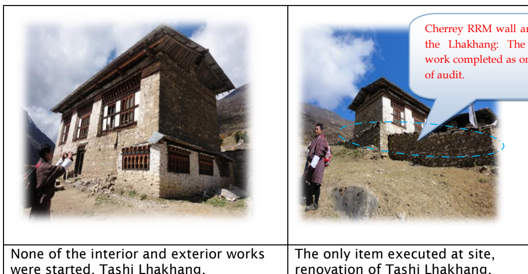
Figure 4.1 Photographs showing poor progress of renovation works
