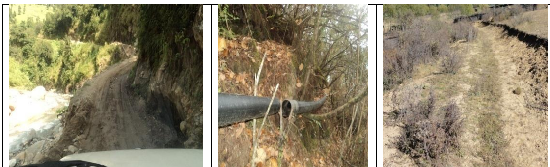
Figure 3.6: Examples of assets created through CDG lacking maintenance
