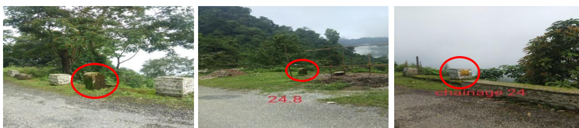
Figure 10: Unsatisfactory road marking works on Gelephu-Trongsa PNH
