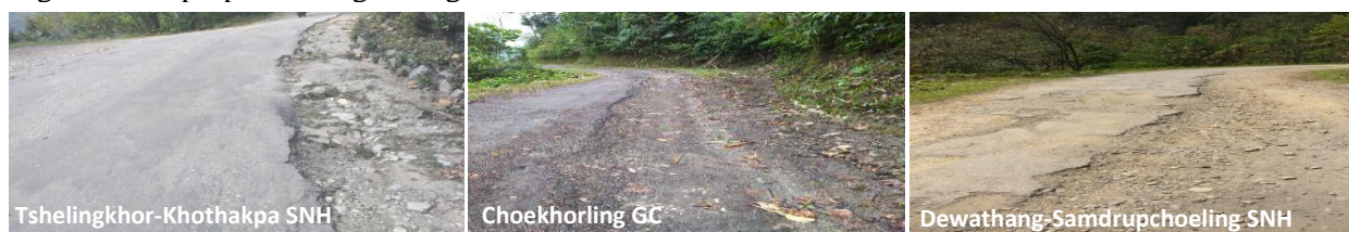
Figure 6: No proper drainage along the roads
