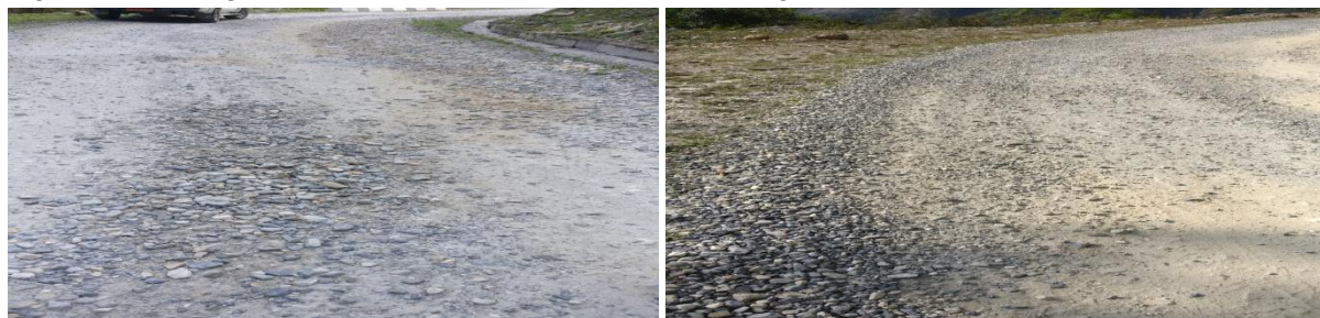
Figure 7: Disintegration of WMM on Tsebar-Mikuri-Durungri SNH
