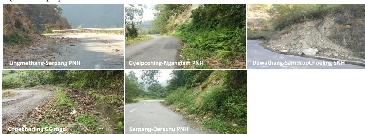
Figure 9: Improper routine maintenance works carried out
