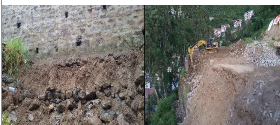
Figure 7: Collapsed wall at Trashigang Middle Secondary School.
