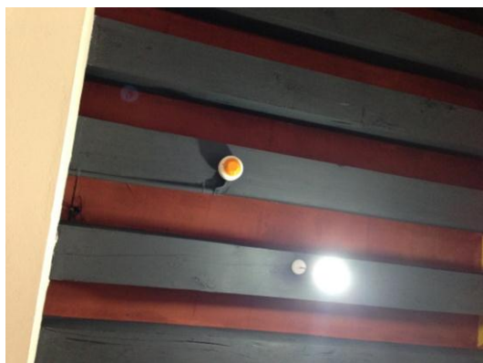
Figure 5: Smoke detector cap not removed
