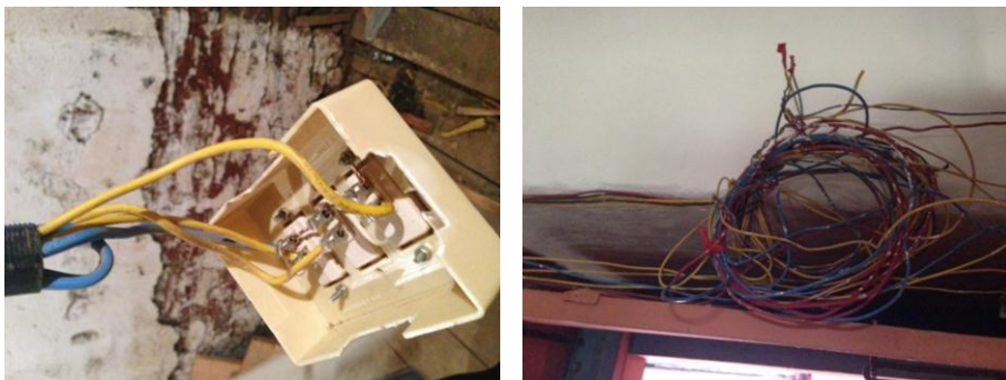
Figure 6: Poor wiring done in Dzongs
