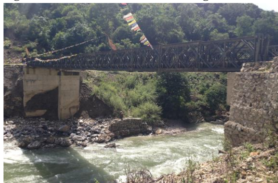
Figure 8: Scoured abutment of Pangzam
