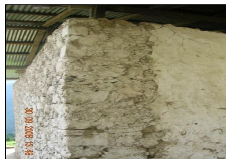
Photograph 4.4(a): The adjacent wall which collapsed several times
