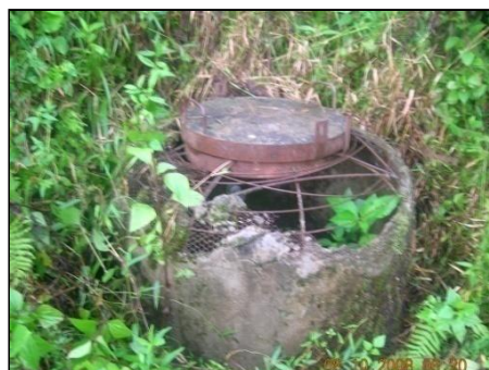
Photograph 4.5 (b): Damaged pressure tank
