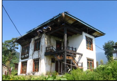
Photograph 4.6 (a): Full view of the Gup office damaged by the storm
