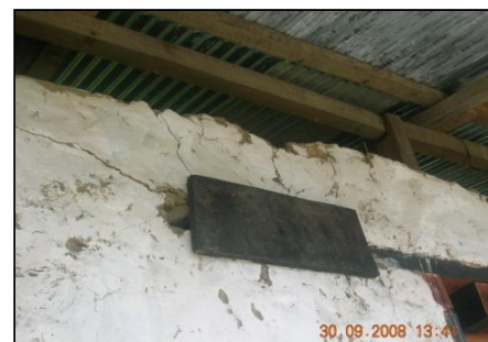
Photograph 4.4(b): Crack developed on the walls
