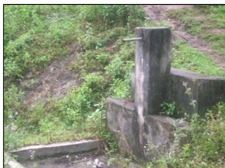
Photograph 4.5 (a): Water Tap near Gup's Office
