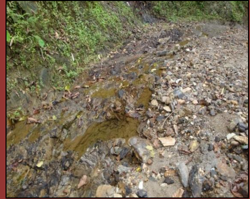
Deorali-chisopani road: Drain gone wrong (Samtse)
