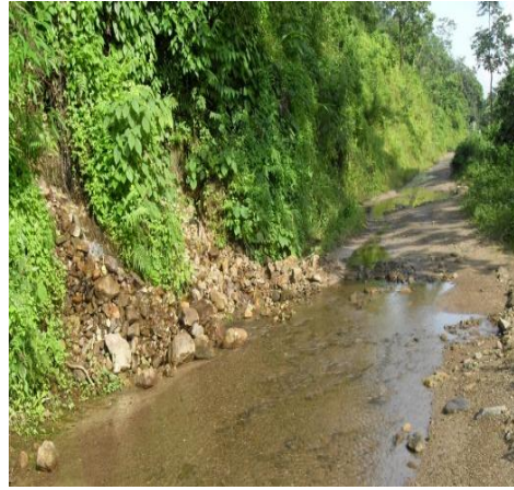
Causeway required Martsalla road (S/Jongkhar)
