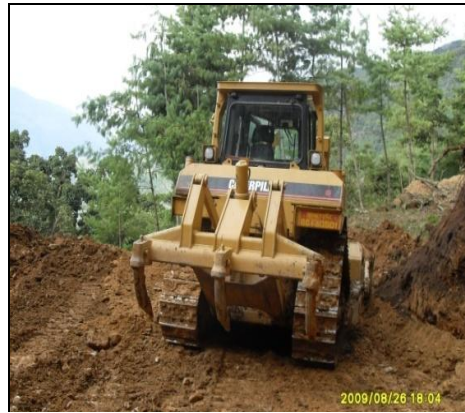
Ramjar farm road constructed only with a bulldozer
