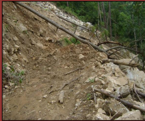
The excavated soil and other materials were dumped over the edge of the roads not adhering to the clauses of the environmental clearances.
