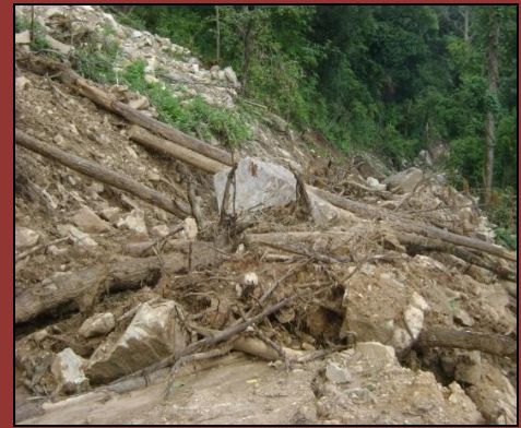
The excavated soil and other materials were dumped over the edge of the roads not adhering to the clauses of the environmental clearances.
