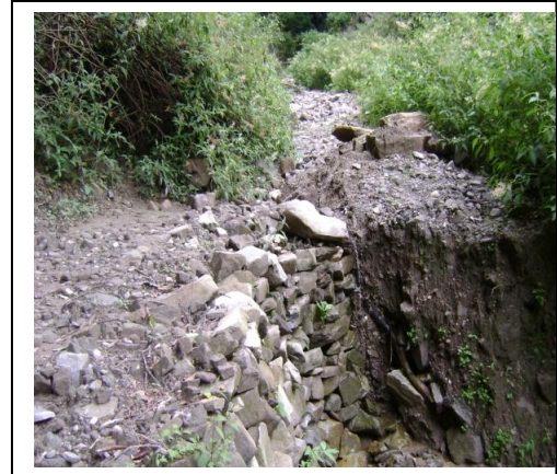
Tshangkha Farm Road, Trongsa
