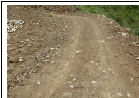
Bidung farm road (Trashigang): high gradient and sharp curves
