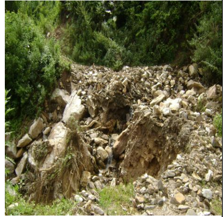
Need for retaining wall. Khagochen road (Dagana)
