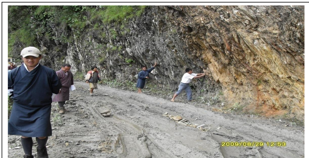
Village workers at the maintenance site in Udzorong farm road, Trashigang
