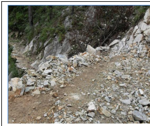
Kalapang- Resa road: ends in a forest (Mongar)
