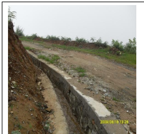
Gonpasingmo-Ngangmalam road (Pemagatshel): Concrete drain provided by DoR
