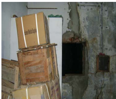
Very poor infrastructure in the interior of the MSD building
