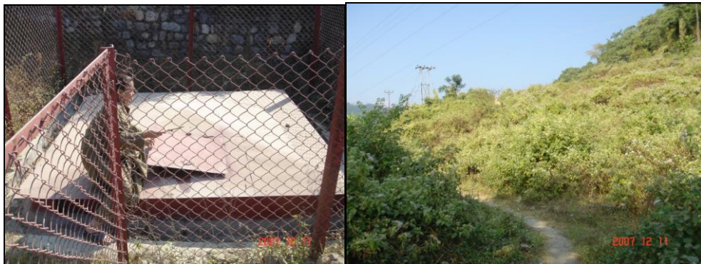
Deep burial pit and waste carrying path leading to the pit.
