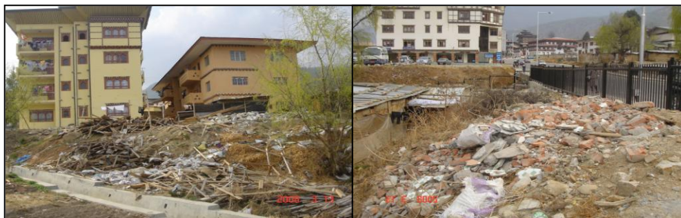
C&D waste lying near the house after construction
