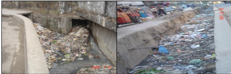
The waste water from neighboring town (Jaigoan) making its way into the storm water drain in Bhutan.
