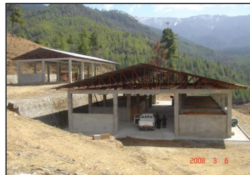
The Compost plant at Serbithang
