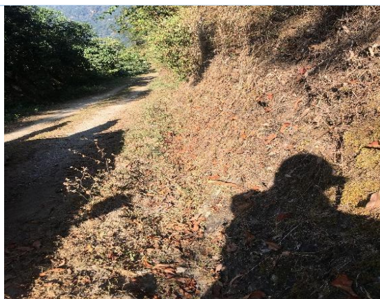
Damji farm road, Bongo, Chhukha. RUG conducted routine maintenance and the farm road was pliable all seasons.
