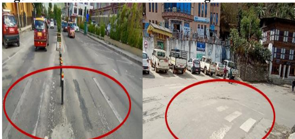
Figure 13: Faded Pedestrian crossings
