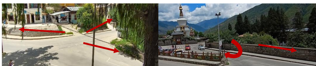
Figure 16: Absence of road markings create confusion and could increase the possibility of accidents
