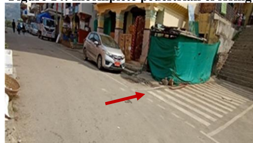
Figure 14: Incomplete pedestrian crossing
