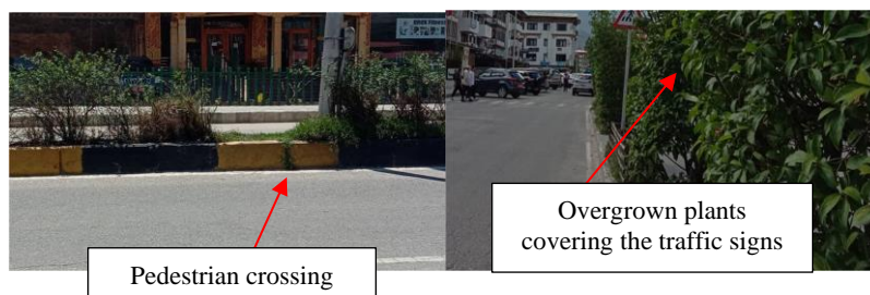
Figure 15: Bushes on road dividers blocking the sight of drivers
