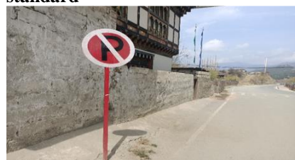
Figure 32: Non-reflective hand painted traffic sign – not as per standard
