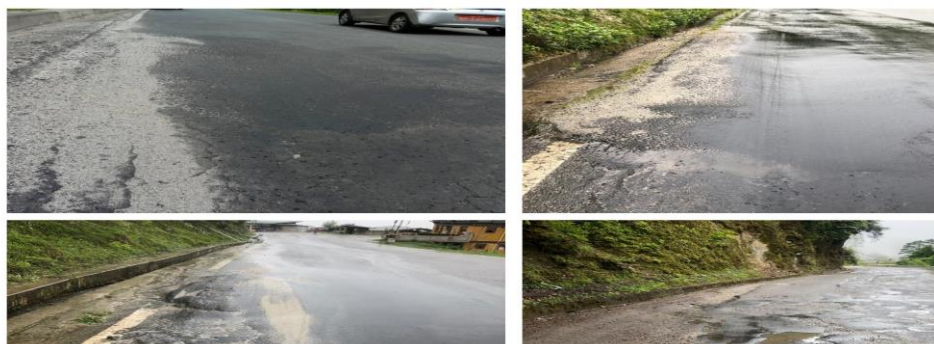
Figure 40: Recessed sections of the road along the Wangdue – Thimphu highway
