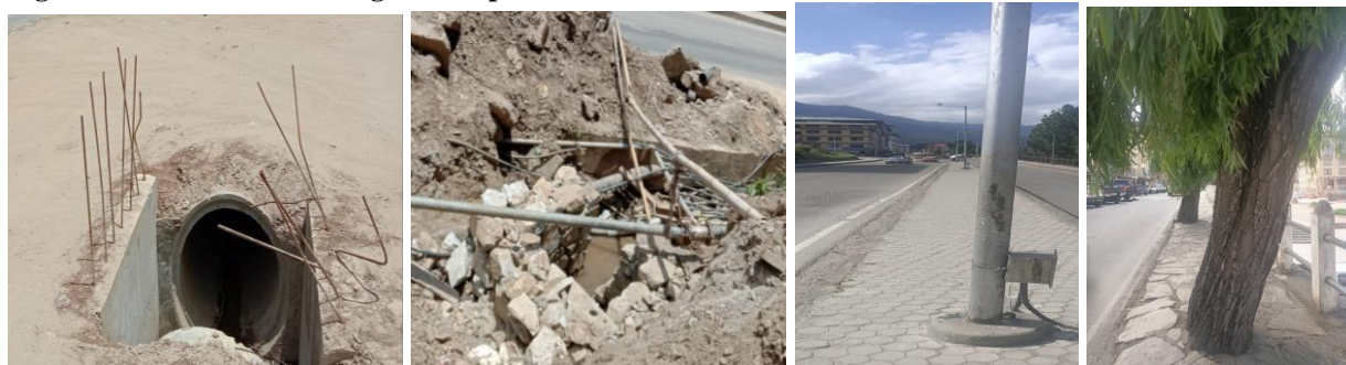
Figure 22: Obstructions along the footpaths
