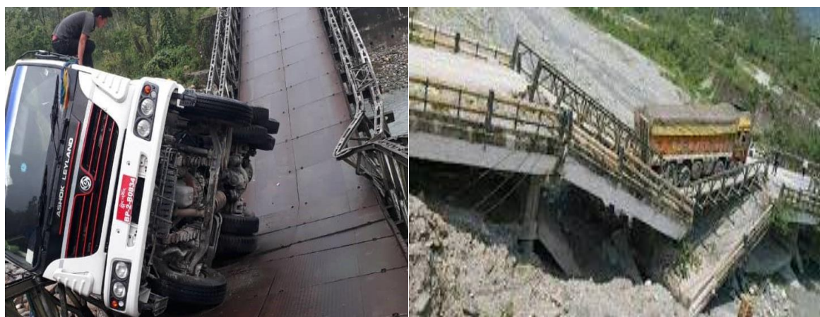
Bailey bridge at Kuchidiana- Samtse
