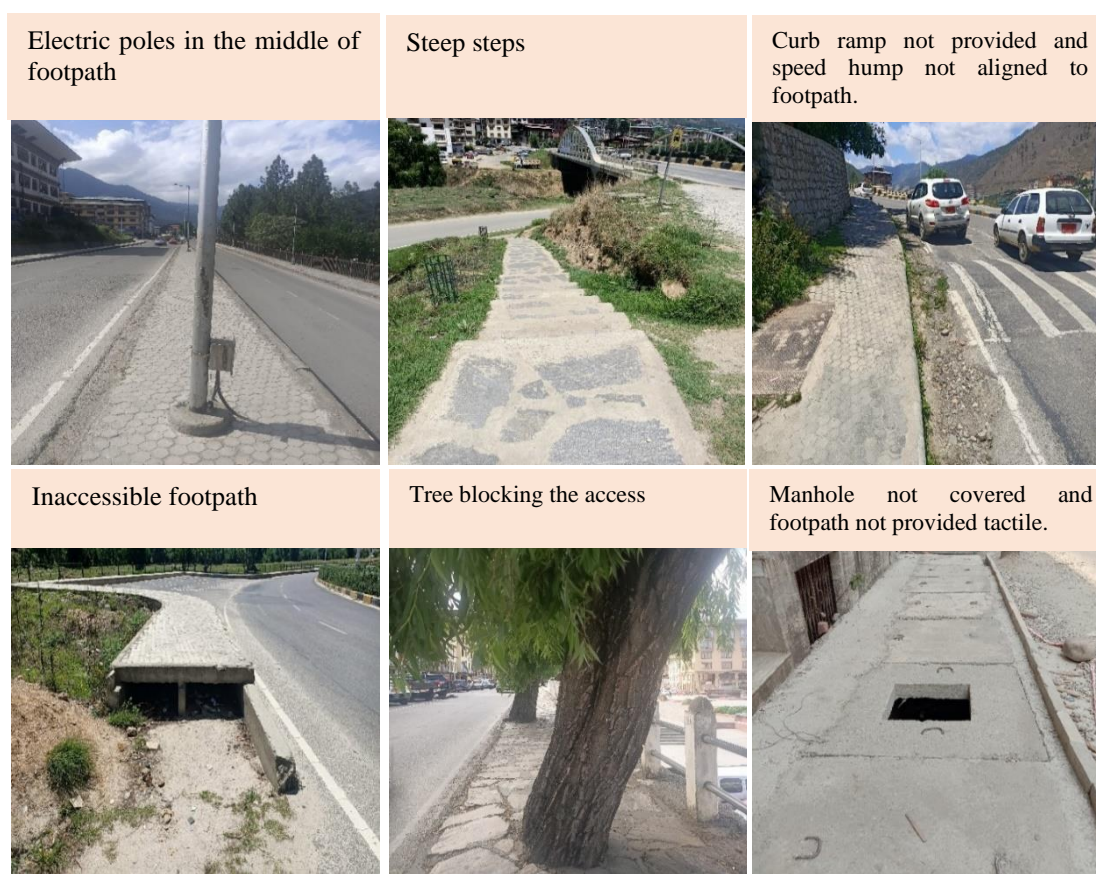
Figure 68: footpaths inhibiting accessibility with reduced mobility of persons with disabilities
