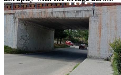
Figure 20: Footpath ending abruptly with the bridge across
