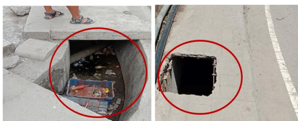
Figure 21: Manholes along the footpaths
