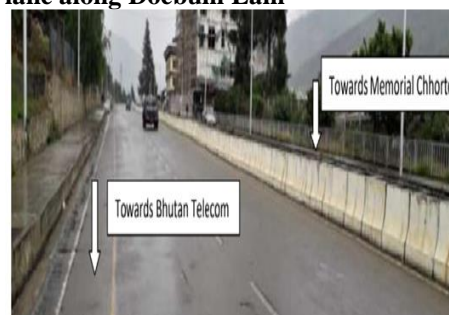
Figure 23: Unsafe and narrow cycling lane along Doebum Lam
