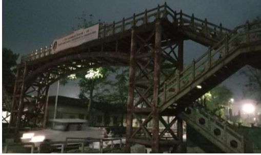
Figure 10: Pedestrian Bridge in Phuentsholing
