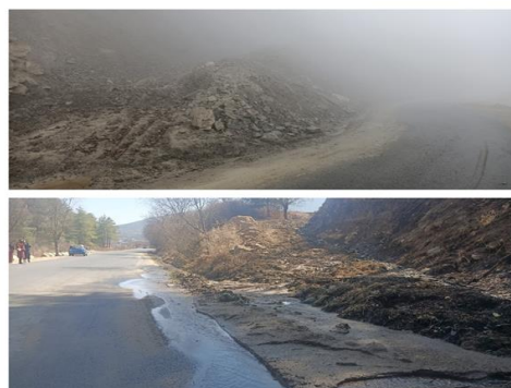
Figure 27: Damages caused by improper access road
