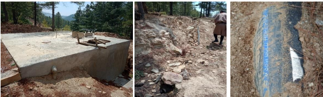
Picture-5: Jalakhar Irrigation Scheme in Chamkhar Throm, Bumthang
