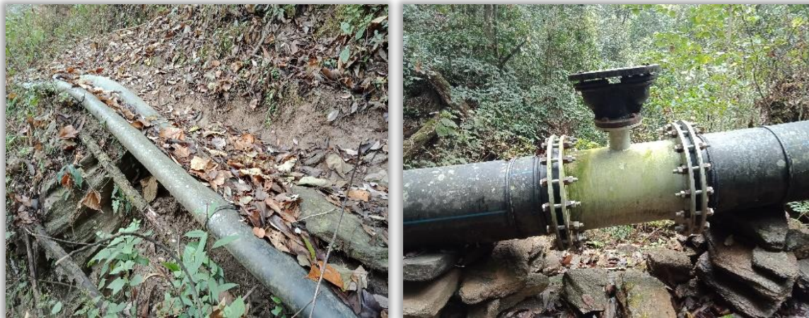
Picture-16: Aum Tshokimo-Wolathang Irrigation Scheme, Toedwang Gewog, Punakha
