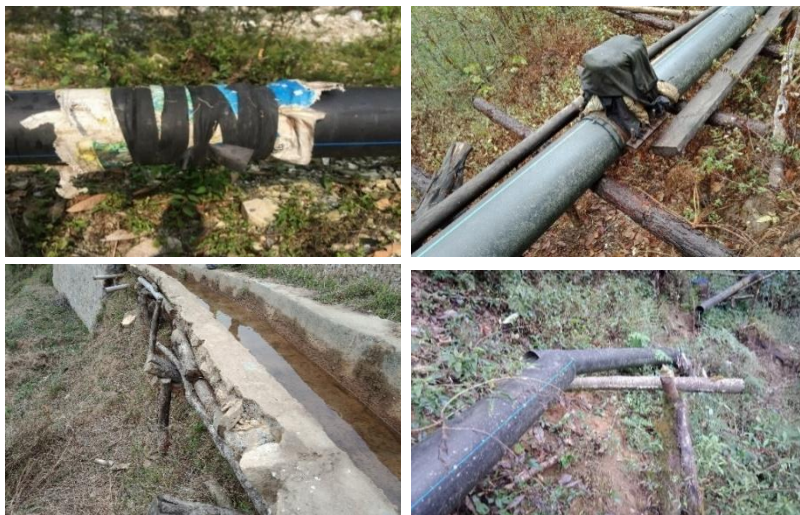
Picture-23: Daba Irrigation Scheme, Nubi Gewog, Trongsa (Top Left); Aum Tshokimo to Wolathang Irrigation scheme, Toedwang Gewog, Punakha (Top Right); Bayul Irrigation Scheme, Dzomi Gewog, Punakha (Bottom Left); Karshong Irrigation Scheme, Nubi Gewog, Trongsa (Bottom Right).
