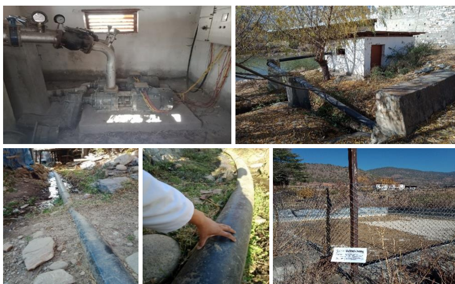
Picture-9: Water Pump system and Reservoir Tank Wangchang Gewog, Paro.
