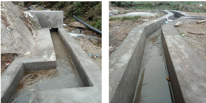
Picture-22: Example of a concrete work executed by the beneficiaries who have skills (Renovation of Jichulum Irrigation Scheme, Kabjisa Gewog, Punakha).
