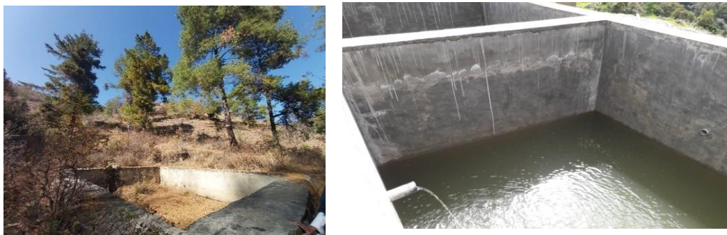
Picture-7: Tserina Reservoir, Sharpa Gewog, Paro (Bottom row left); erstwhile reservoir in Threlphu, Kangpara Gewog, Trashigang (Bottom Row Right).
