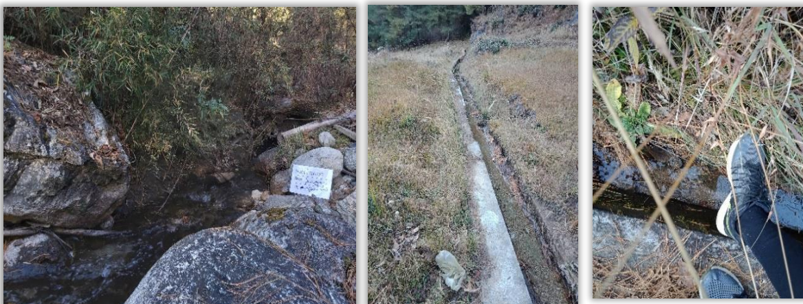
Picture-14: Janagakha-Phongdho Irrigation Scheme, Tsento Gewog, Paro
