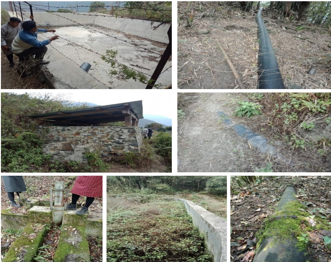
Picture-6: Monmogang Reservoirs and Irrigation facilities, Korphu Gewog, Trongsa (Top two Rows); Mang Gi Zing, Talo Gewog, Punakha (Bottom Row)
