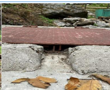
Image 5: Opening without provision for locking, and openings on top of the sediments
