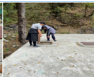
Image 5: Opening without provision for locking, and openings on top of the sediments
