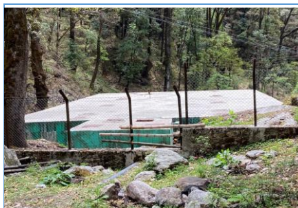
Image 4: Entry point to the sedimentation tank with bamboo pole fencing.
