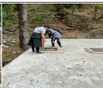
Image 5: Opening without provision for locking, and openings on top of the sediments.
