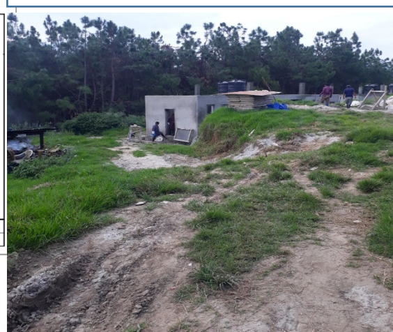
Figure 3.16: Construction of toilet without access by ramp or footpath
