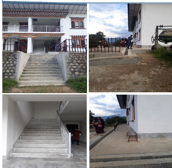
Figure 3.14: Inaccessible ramps constructed after the drainage, no ramps to access the first floor of the building
