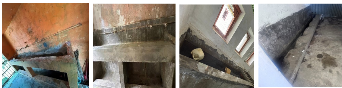
Figure 11: Worn out common wash basin and urinals on the floor
