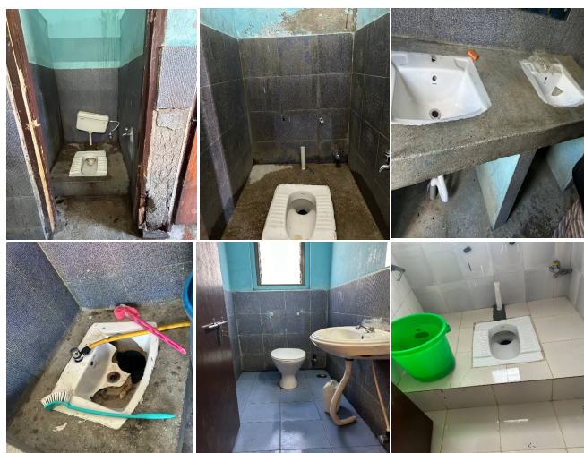
Figure 13: Non-functional flushes and damaged sinks
