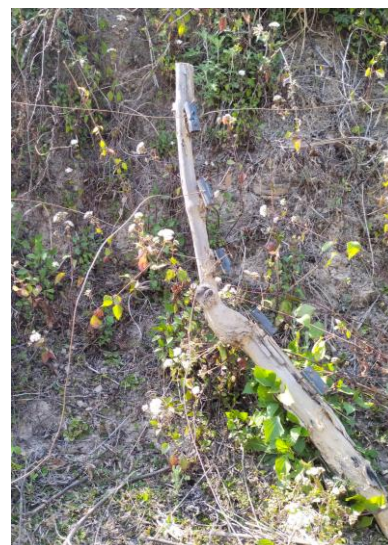
Fallen wooden post with disconnected wires causing power loss to the entire fence, allowing animals to pass through.
