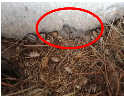
Example of a cemented feeding trough with a worn-out base, about which farmers complain about a risk of cement ingestion.
