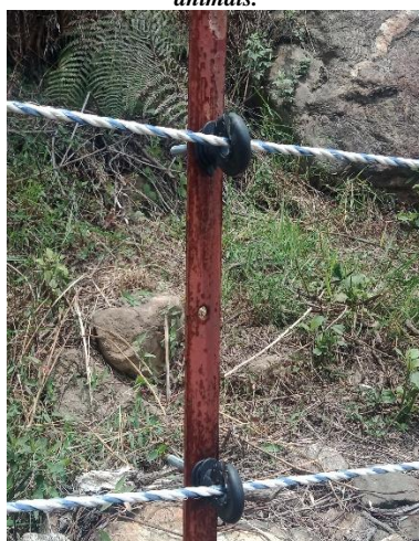
Example of a potential innovation: electric fence using iron posts and wires reinforced with nylon rope (not supported by CARLEP).
