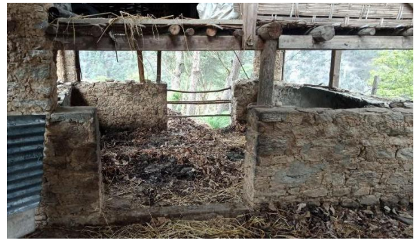
Cattle shed not complying the standard design and concrete flooring (CARLEP support: cement, cow mat and CGI sheets)
