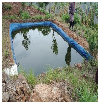
Example case from Yangneer Gewog, Trashigang, representing a typical plastic pit developed under CARLEP's support to store water for orchard and kitchen garden (example of a best practices to replicate in other places).
