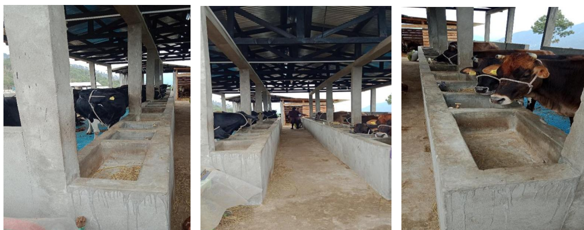
Interior design of the Cattle Shed: double-row face-to-face stall layout with concretasied feeding trough
