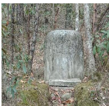
Several distribution tanks installed at strategic locations to distribute the water to surrounding fields (Chhali Gewog, Mongar)
