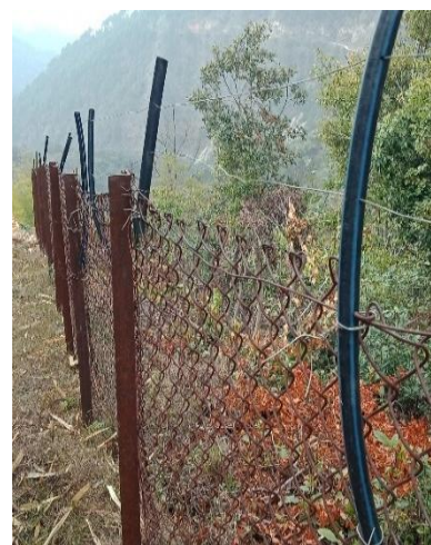
Example of a potential innovation: a hybrid chainlink and electric fence, known to protect against monkeys (piloted at ARDC-Wengkhar; not supported by CARLEP).
