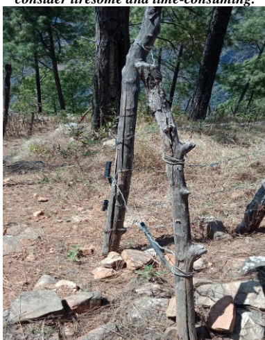
Typical example of an electric fence with worn-out wires replaced by barbed wire.
