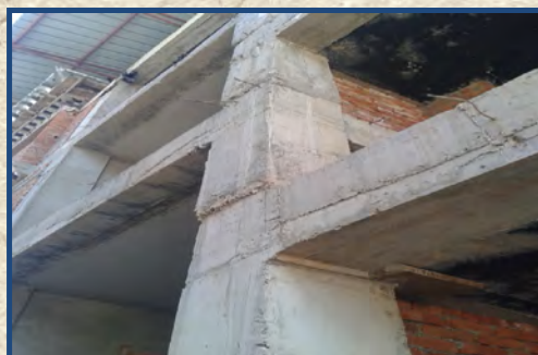
Fig 5.2: Defective alignment of beams
