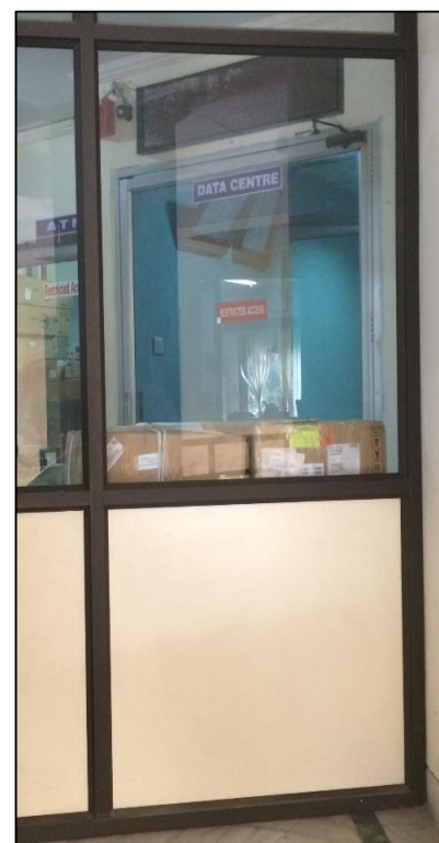
Figure 3: Non-laminated glass partition in front of Data Centre door
