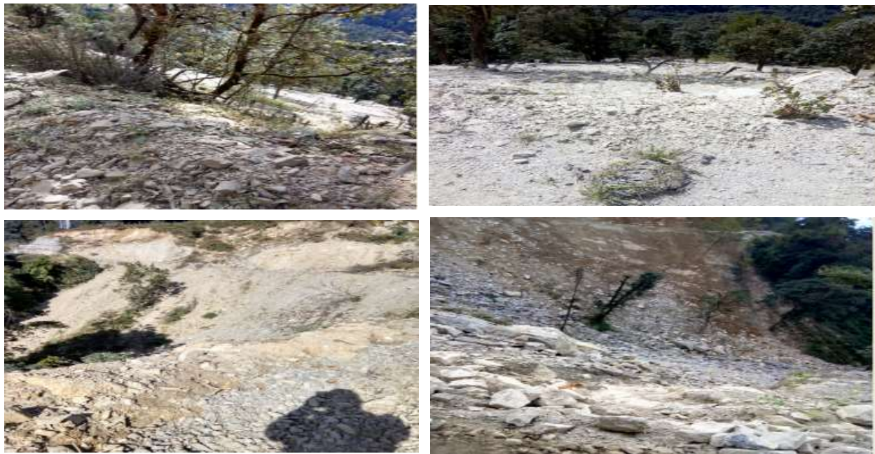
Fig: 2.17.10-Spoil materials dumped and freely rolled/pushed over the hill causing damaged to the environment
