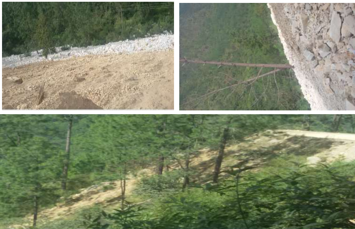
Fig.: 2.17.14- Freely rolled/pushed down of excavated materials over the hill
