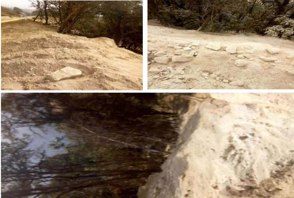
Fig: 2.17.6-Spoil materials dumped and freely rolled/pushed over the hill causing damaged to the
