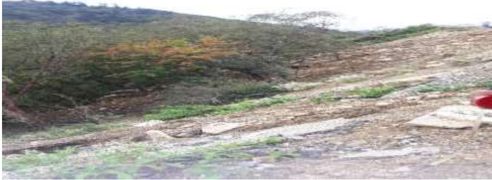
Fig: 2.17.1- Spoil materials rolled down the cliff in places other than designated
