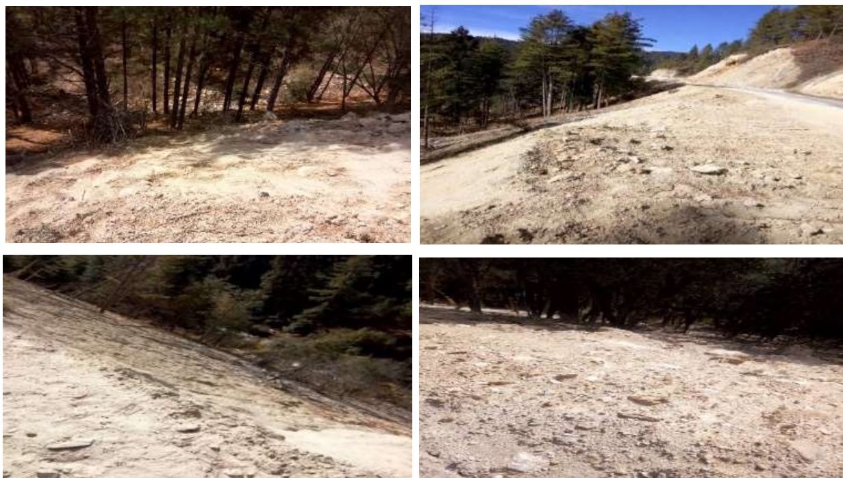
Fig: 2.17.9-Spoil materials dumped and freely rolled/pushed over the hill causing damaged to the environment
