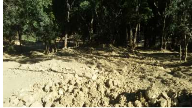
Fig: 2.17.12- Freely rolled/pushed down of excavated materials over the hill
