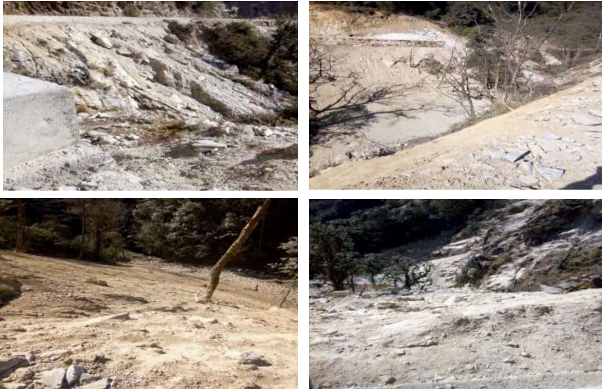
Fig: 2.17.2-Spoil materials dumped and freely rolled/pushed over the hill causing damaged to the environment
