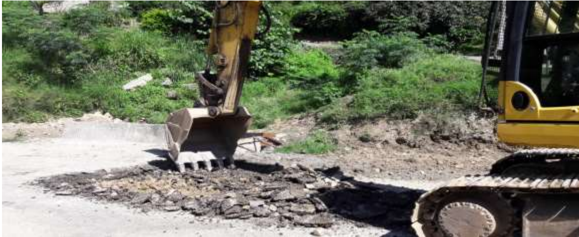
Response to Para 7.1: Complete stripping of existing bituminous in progress
