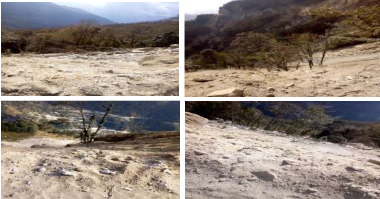
Fig: 2.17.3- Spoil materials dumped and freely rolled/pushed over the hill causing damaged to the environment
