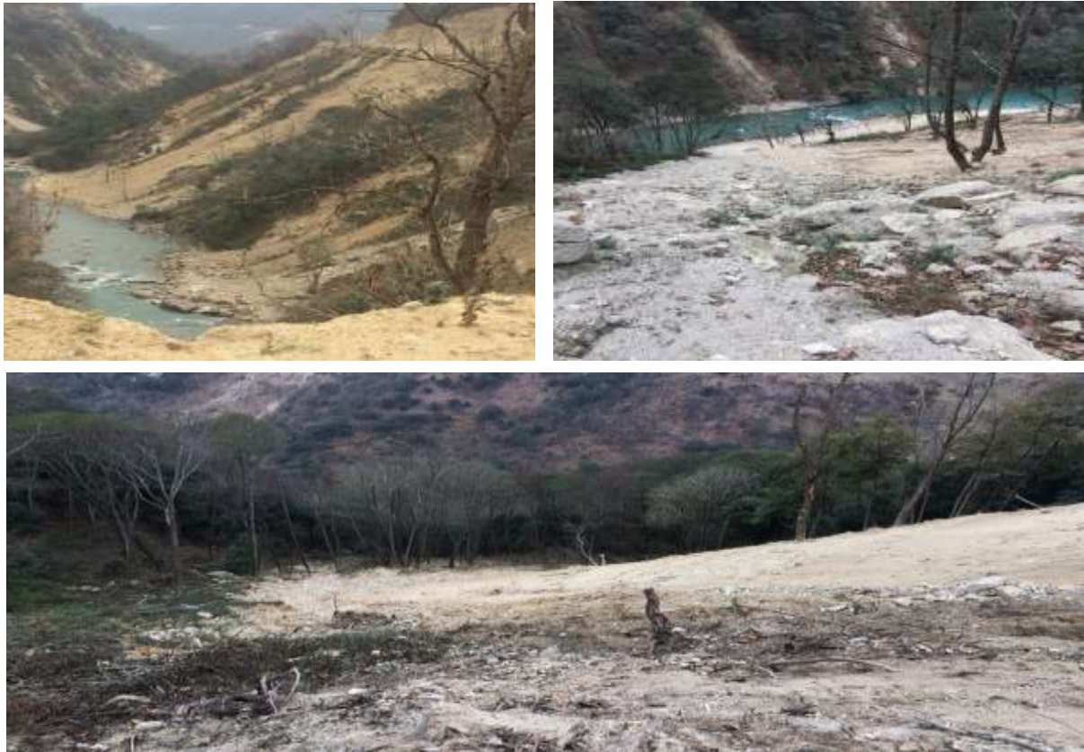
Fig: 2.17.4- Spoil materials dumped and freely rolled/pushed over the hill causing damaged to the environment
