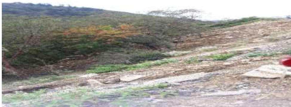
Fig: 2.17.1- Spoil materials rolled down the cliff in places other than designated areas
