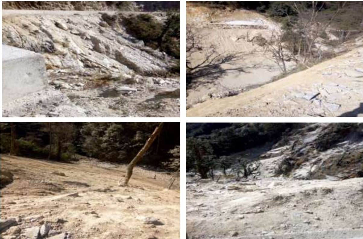
Fig: 2.17.2-Spoil materials dumped and freely rolled/pushed over the hill causing damaged to the environment
