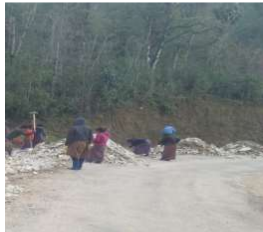
Response Para 21.2: Breaking the materials to required sizes
