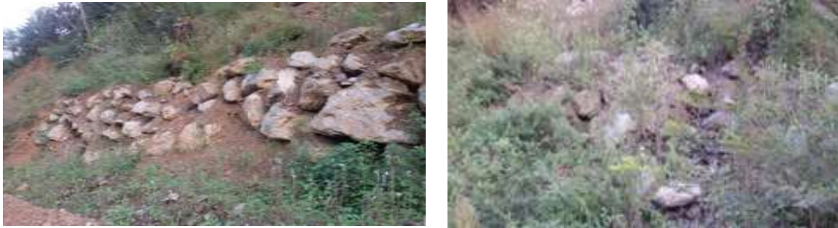
Fig: 23.1: Damaged boulder barriers
