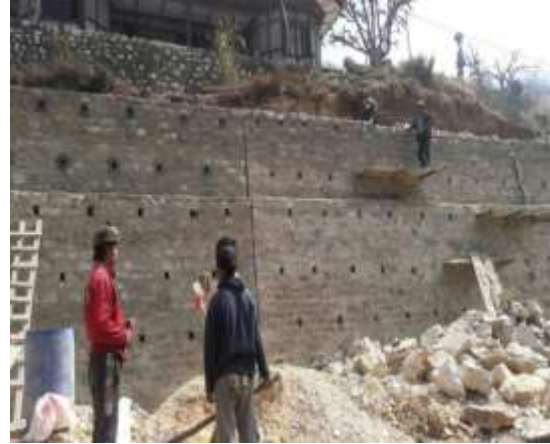
Response to Para 4.6- defective RRM Walls
