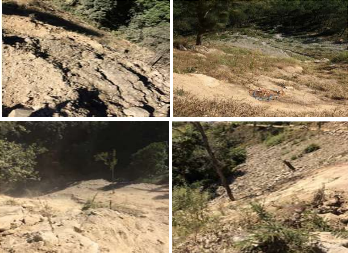
Fig: 2.17.16-Freely rolled/pushed down of excavated materials over the hill
