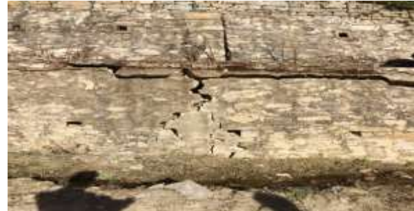
Fig: 3.2(1)- Damaged RRM
