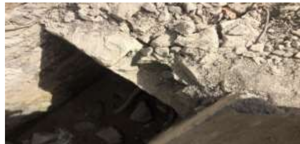
Fig: 3.2(1)- Damaged RRM
