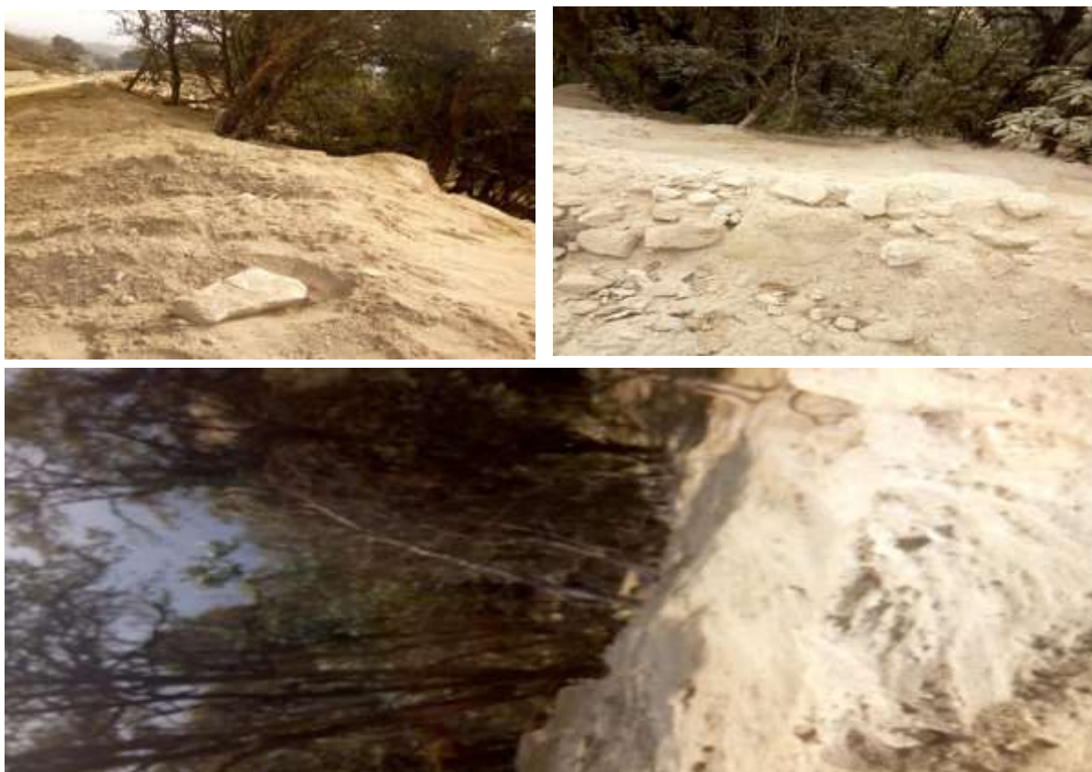
Fig: 2.17.6-Spoil materials dumped and freely rolled/pushed over the hill causing damaged to the environment
