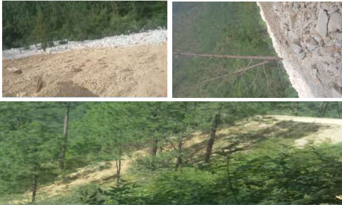
Fig.: 2.17.14- Freely rolled/pushed down of excavated materials over the hill
