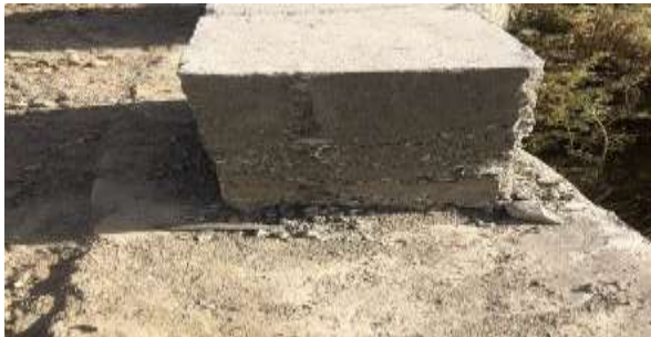
Fig: 3.2- Parapets with honey comb
