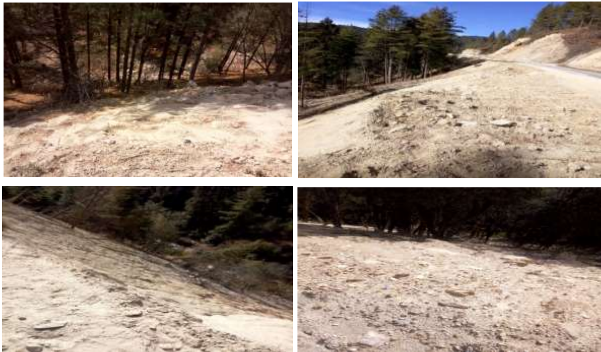
Fig: 2.17.9-Spoil materials dumped and freely rolled/pushed over the hill causing damaged to the environment
