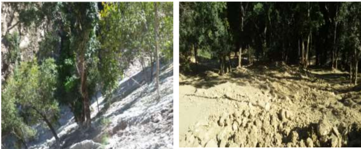
Fig: 2.17.12- Freely rolled/pushed down of excavated materials over the hill
