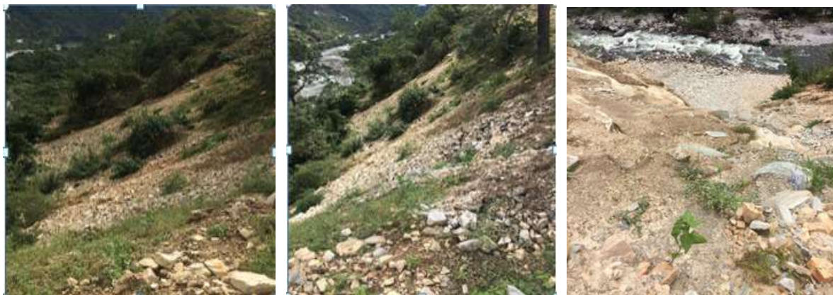
Fig: 2.17.15-Roll over of mucks over the valley
