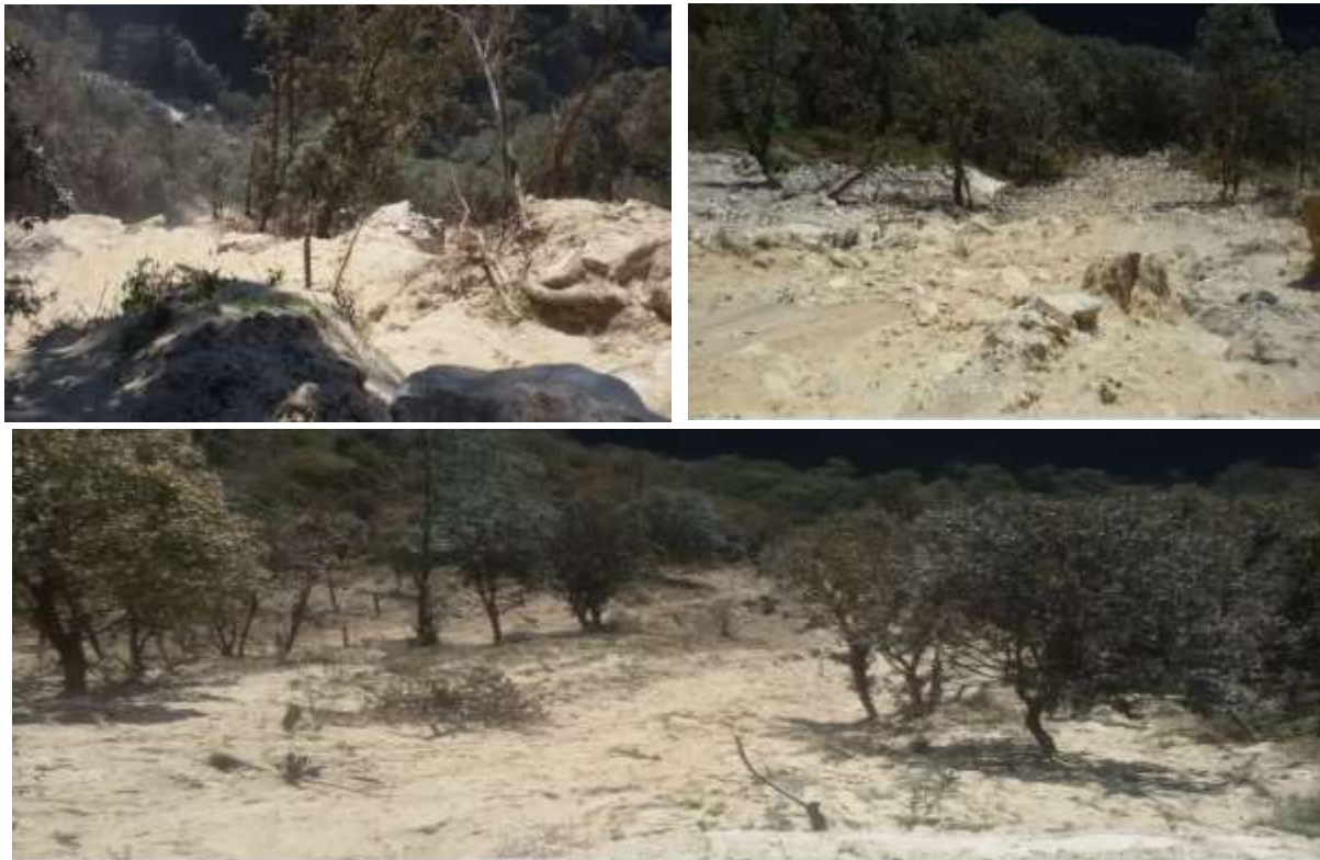
Fig: 2.17.5-Roll over of mucks over the valley
