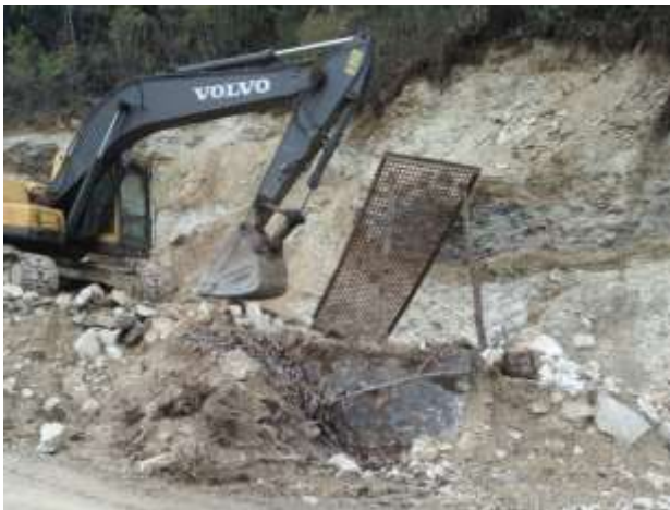
Response Para 21.2: Screening the materials
