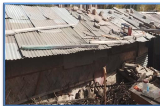
Temporary roofing in Changidphu
