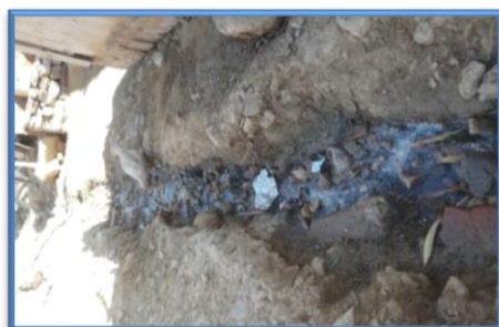
Waste water flowing in open space
