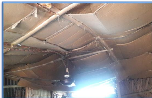
Ceiling made of waste cardboard boxes
