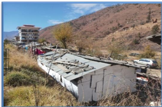
Roof material, below Babesa High way
