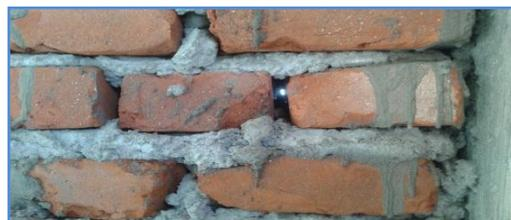
Motor applied too thick showing poor workmanship.
