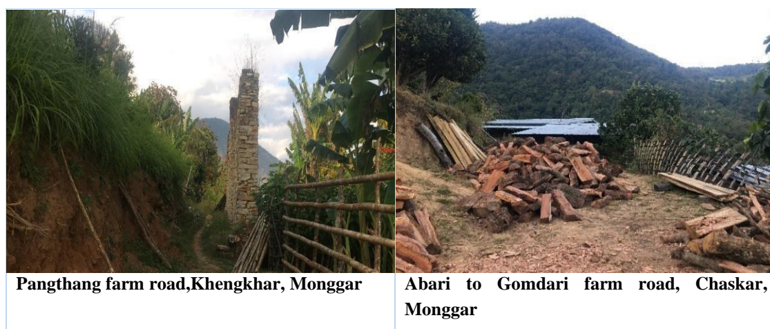
Figure 3.6: Land not provided during construction although it was agreed initially
