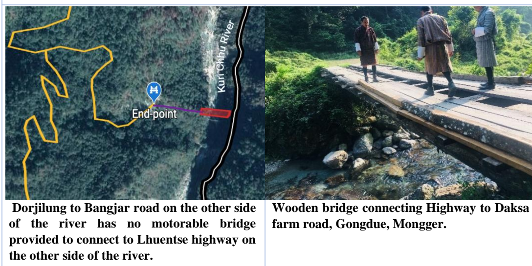
Figure 3.4: Roads without provision of permanent bridges
