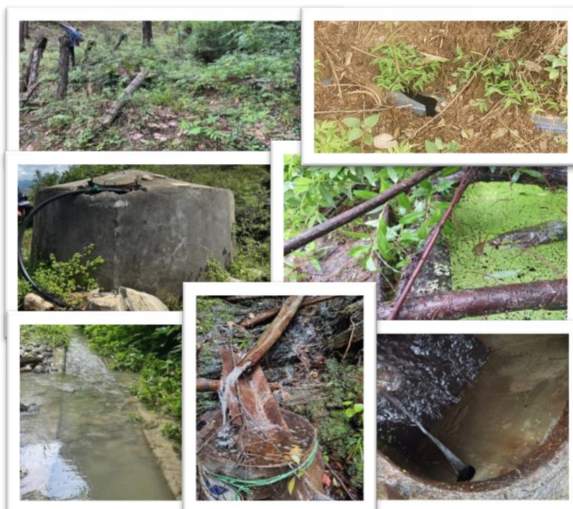
Figure 14: Lack of adequate O&M activities
